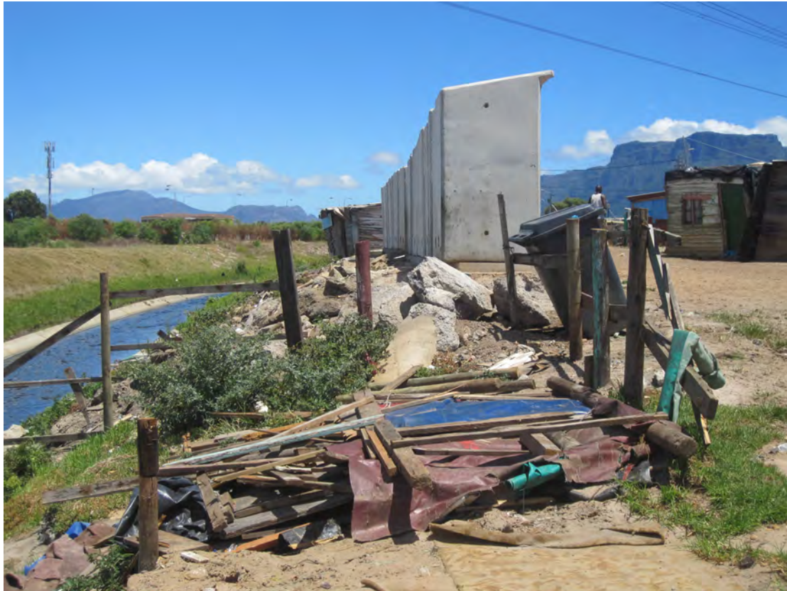
Photo 2: Communal toilets and waste dumping in Joe Slovo. Source: Author.
