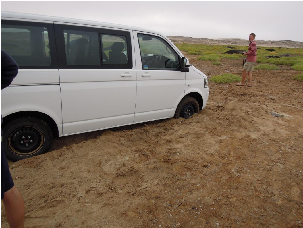
Figure 111 Sand in the drainage channels. A likely source of saltators.
