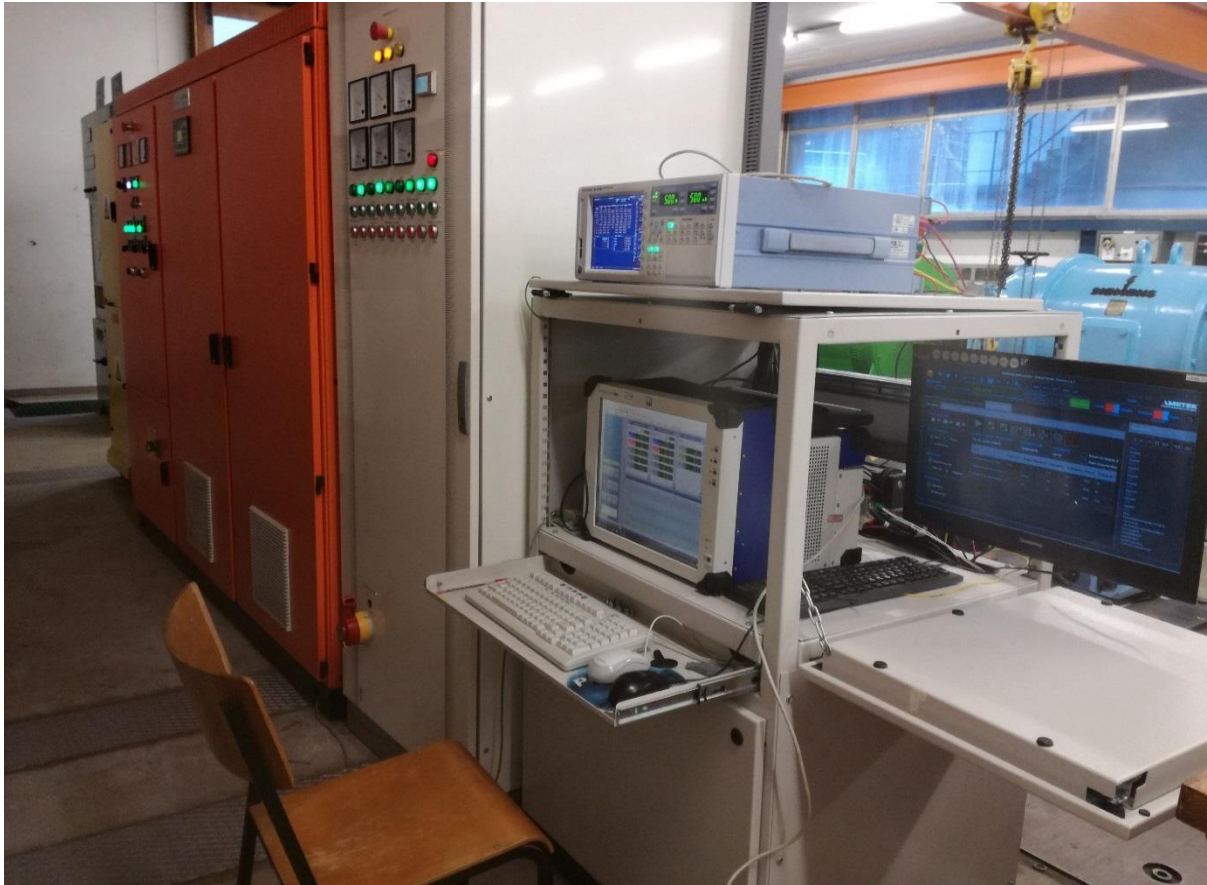
Fig.5.3 Laboratory test bench showing DAQ (right), Drive panel (orange) and supply change-over panel (white)
