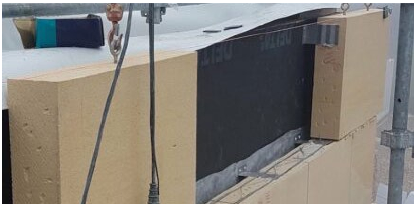
Figure 78 Studiolada healthcare centre assembly of limestone blocks for facade
