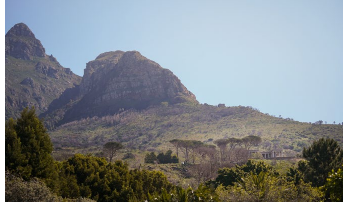
Figure 22 Rhodes Memorial on the foot of Devil's Peak visible from far distances across the city
