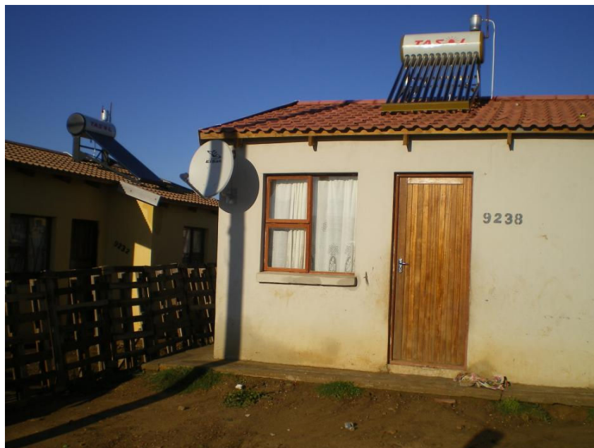
Figure 11: Solar water heaters installed in Zanemvula
