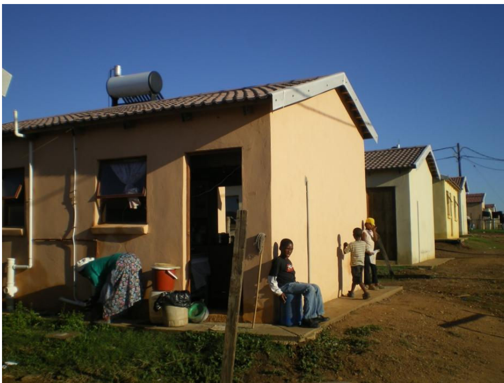
RDP housing in Zanemvula after the implementation of the municipal solar water heater roll-out
