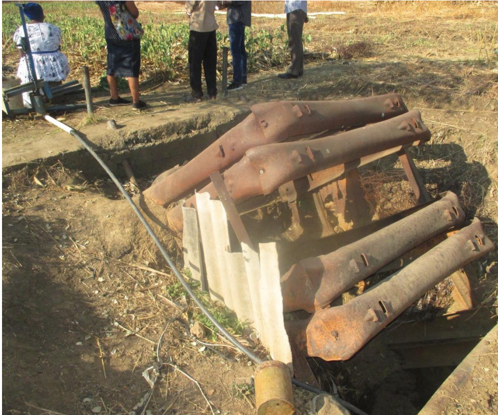
Figure 5.15: Connection from the well to the treadle pump.
