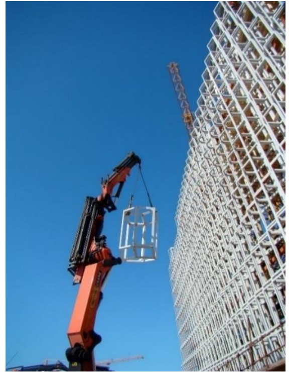
Figure 30. Assembly of façade (Source: Osbjørn Jacobsen, 2011)
