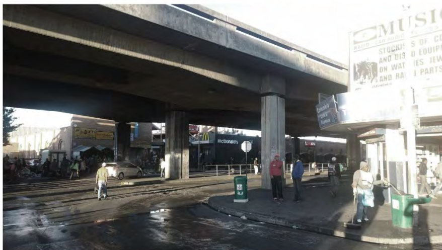
16. TIENIE MEYER ELEVATED HIGHWAY
