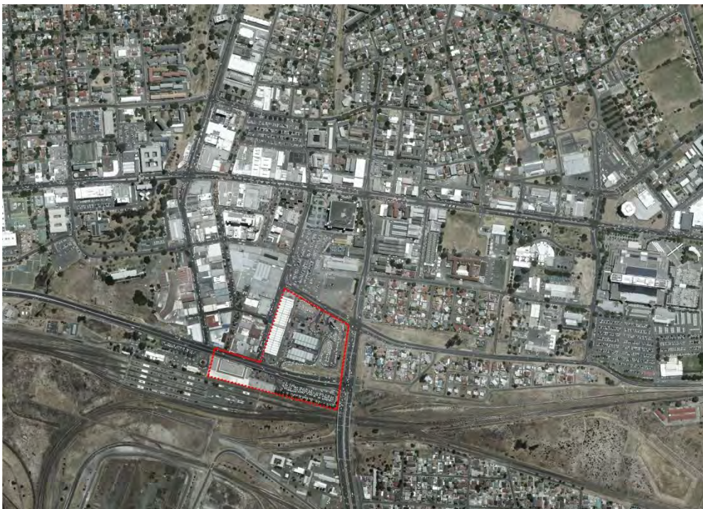
12. CONTEXT PHOTO: Bellville Public Transport Interchange precinct
