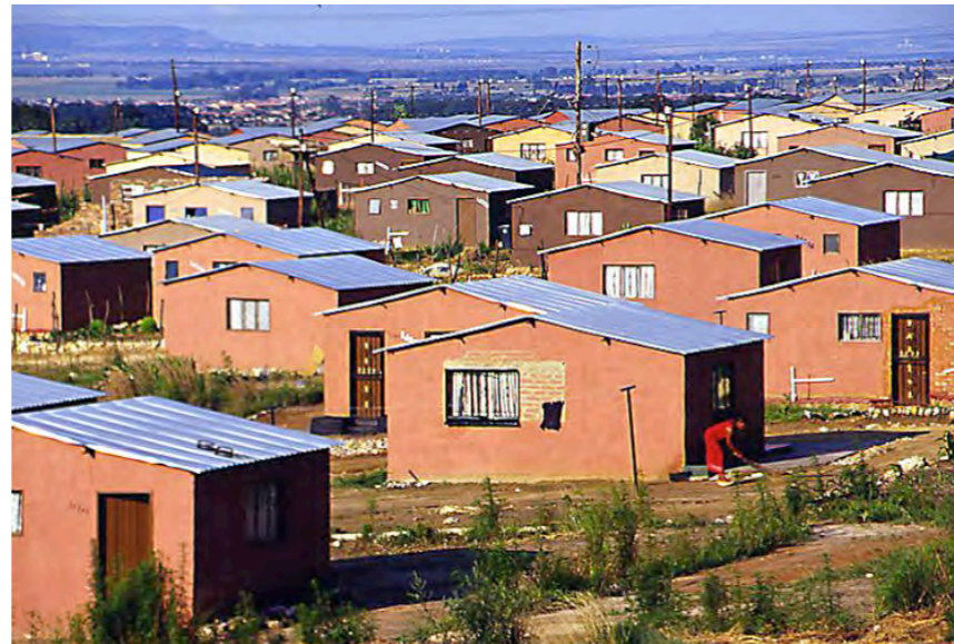
Figure 14: Individual dwelling units/Free-standing, single storey units on the Cape Flats in Cape Town characterize the generic approach to low-cost housing developments (Source: http://www.livingneighborhoods.org ).
