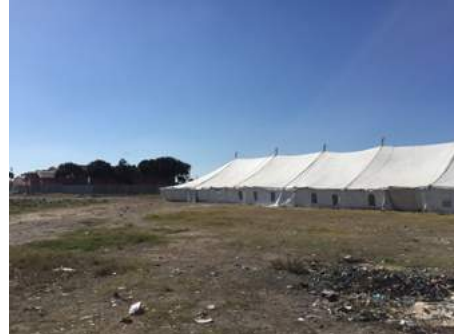
Image indicating the scale of the tent structure
