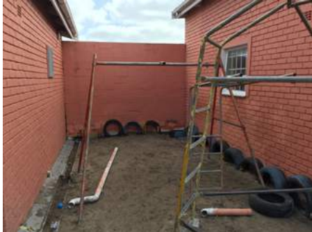
Damaged and insufficient play space at the ECD
