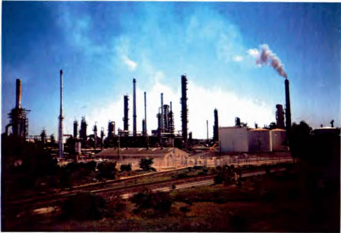
Figure 3. View of Caltex oil refinery releasing pollutants into the atmosphere from raised stacks.
