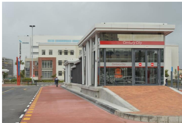
Figure 4: MyCiTi closed station (source Futurecapetown.com)
