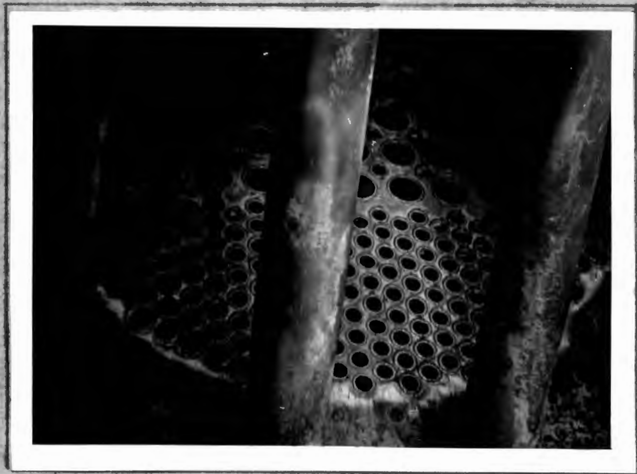
A CLEAN FIREBOX TUBEPLATE.
