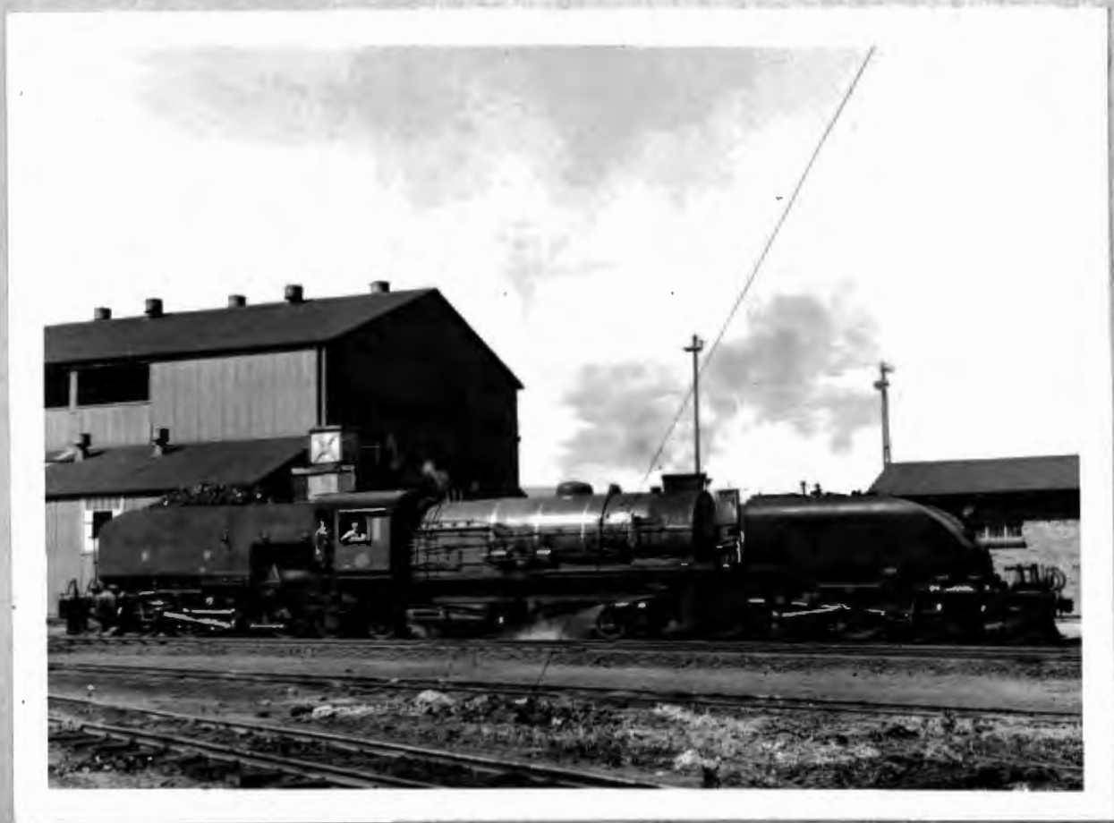
ENGINE No. 380 FITTED WITH GIESL EJECTOR.
