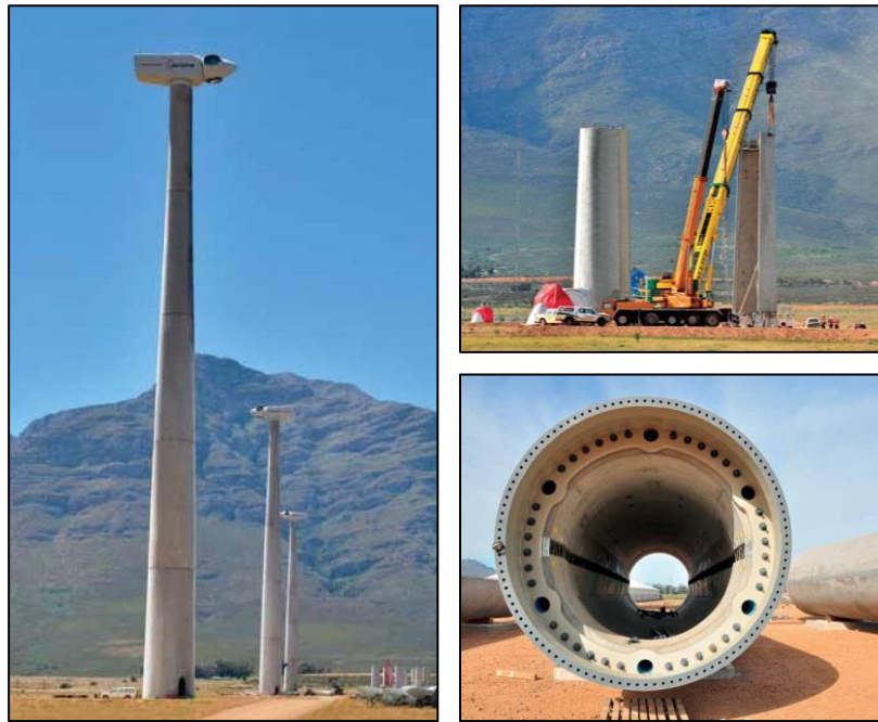
Figure 2.8: Precast concrete towers at the Gouda Wind Farm
