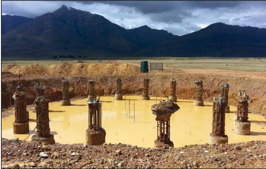
Figure 2.12: Piling completed for a tower base at the Gouda Wind Farm
