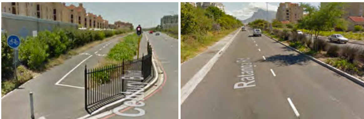
Figure 5.26: Ratanga Road NMT infrastructure (Source: Google Street View)
