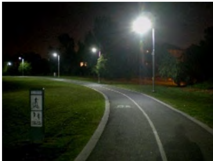
Figure 6.11: Well-lit NMT infrastructure (Source: Bicycle Network Australia, 2015)
