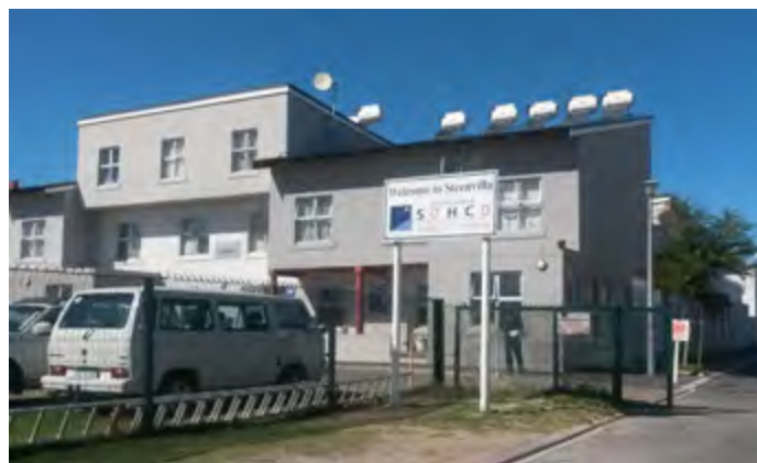
Figure 6.4: Steen Villa social housing project (Source SOHCO, 2015)
