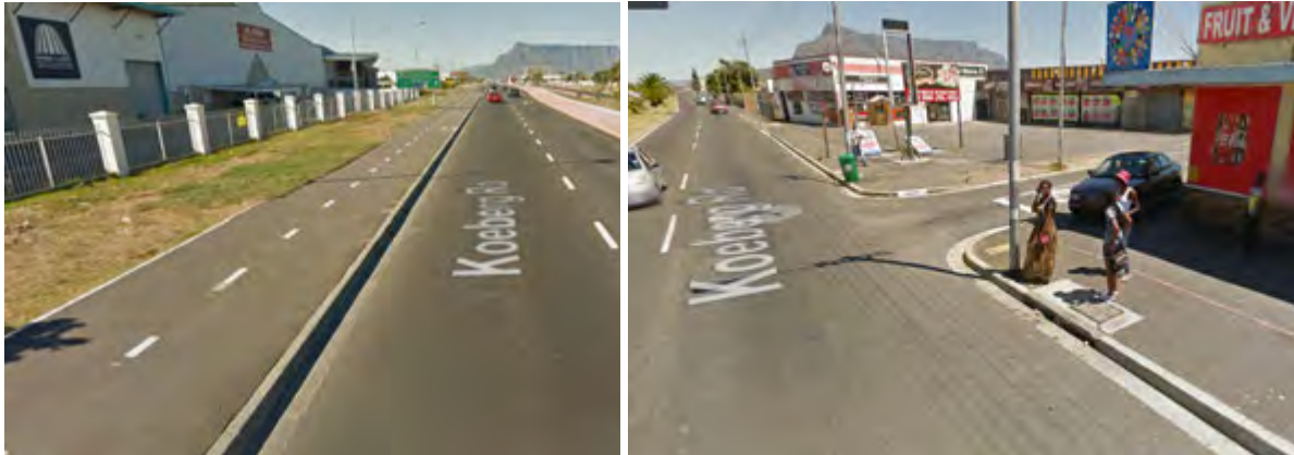
Figure 5.17: Koeberg Road NMT infrastructure (Source: Google Street View)
