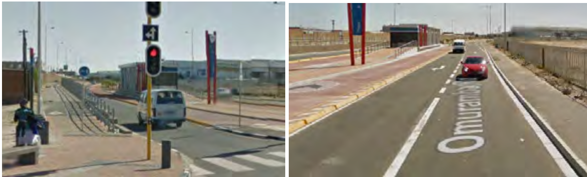
Figure 5.25: Omuramba Road NMT infrastructure (Source: Google Street View)
