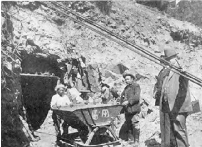
The removal of excess matter form the horizontal service audit.
