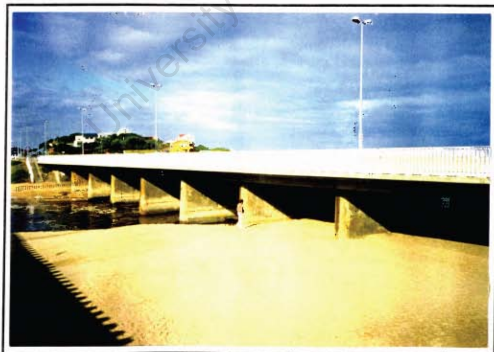
Figure 5.10: Touw River Bridge, Wilderness
