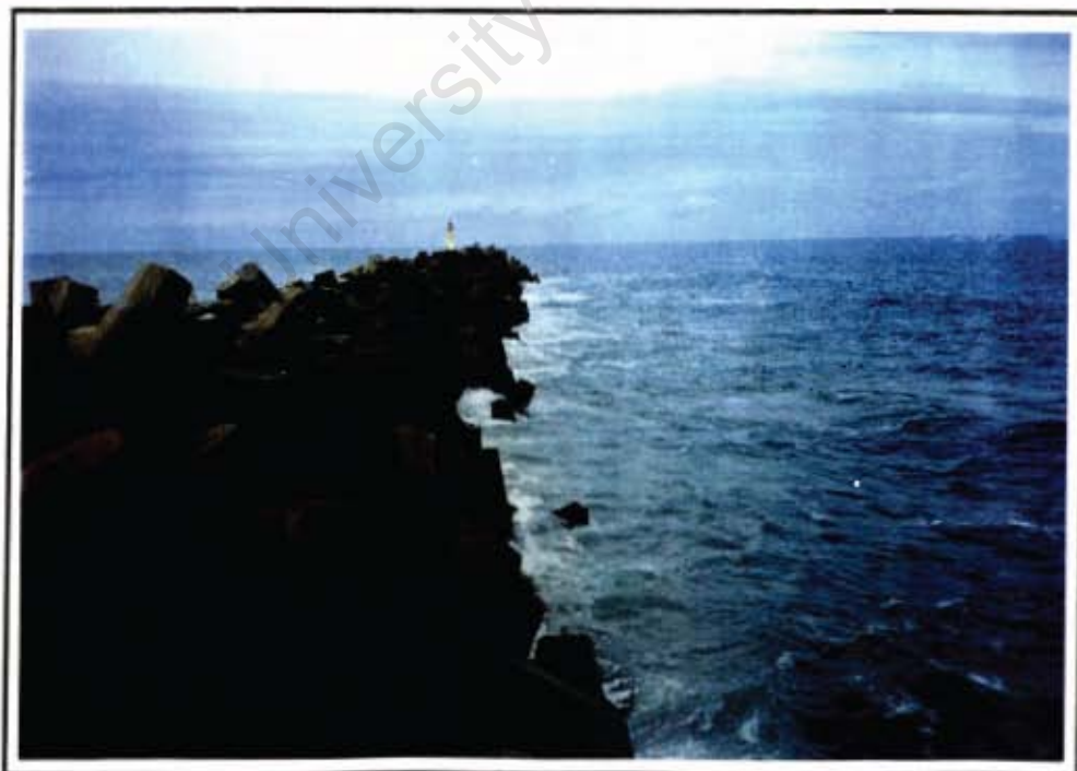
Figure 5.8: East London Breakwater
