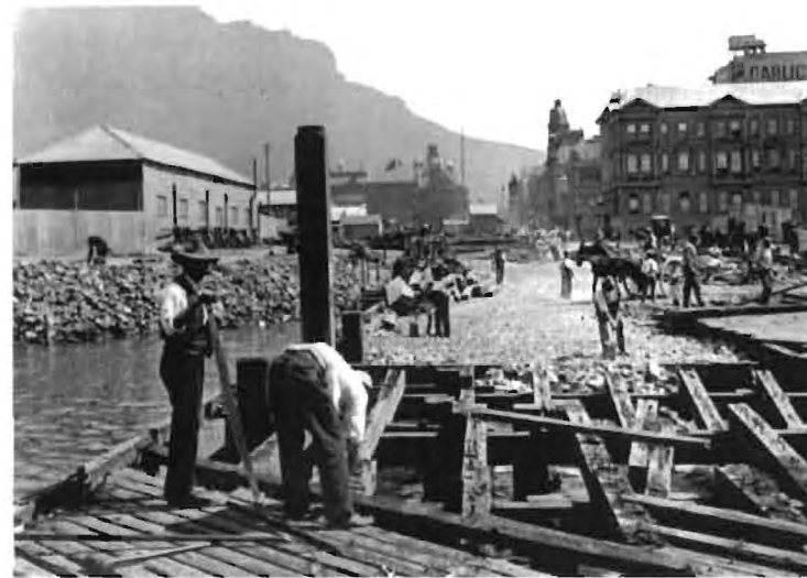
breaking up of the old Pier, 1940
