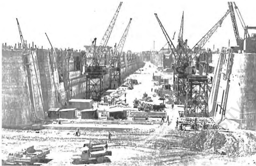
Figure 12 Construction of the Table Bay Harbour
