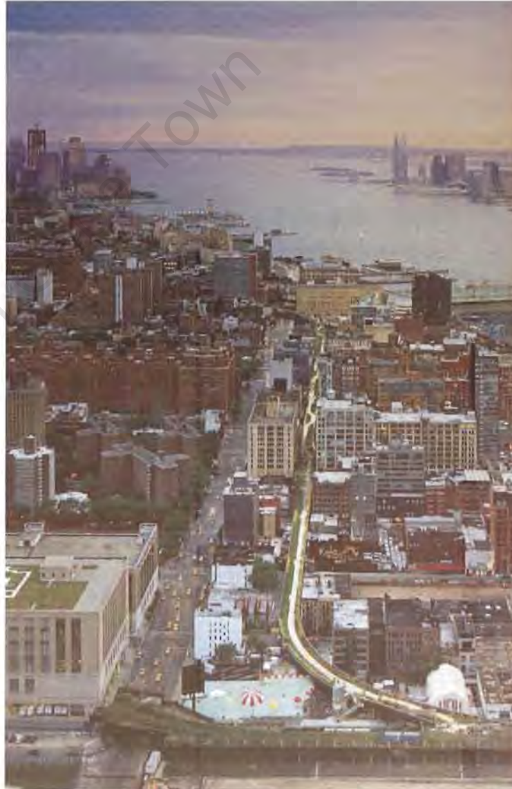
Figure 32 Left: Aerial view on The Highline Park in New York, Opposite: elevated industrial artefact
