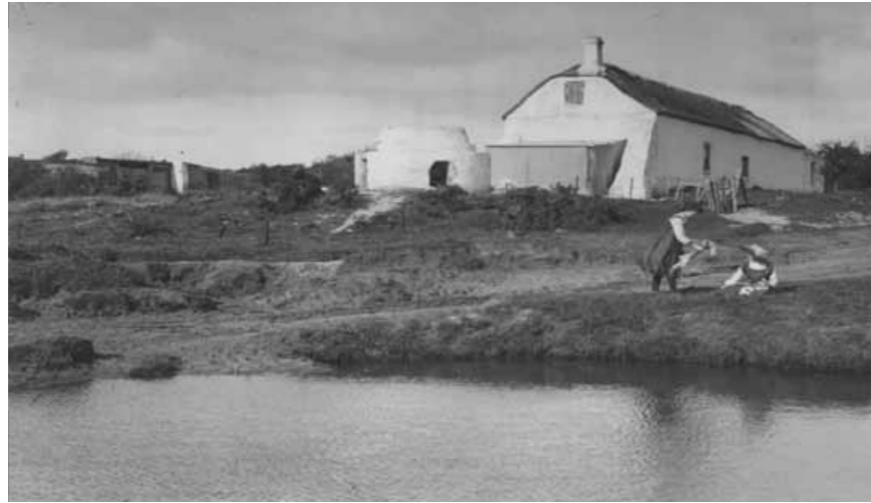
fig. 8. Klein Zoar, the historic cottage on the edge of the vlei, built in 1710 and reputedly the home of folk hero Wolraad Woltemade. It was originally separated from Paarden Eiland by a wide stretch of water, where fish were caught on a daily basis.
