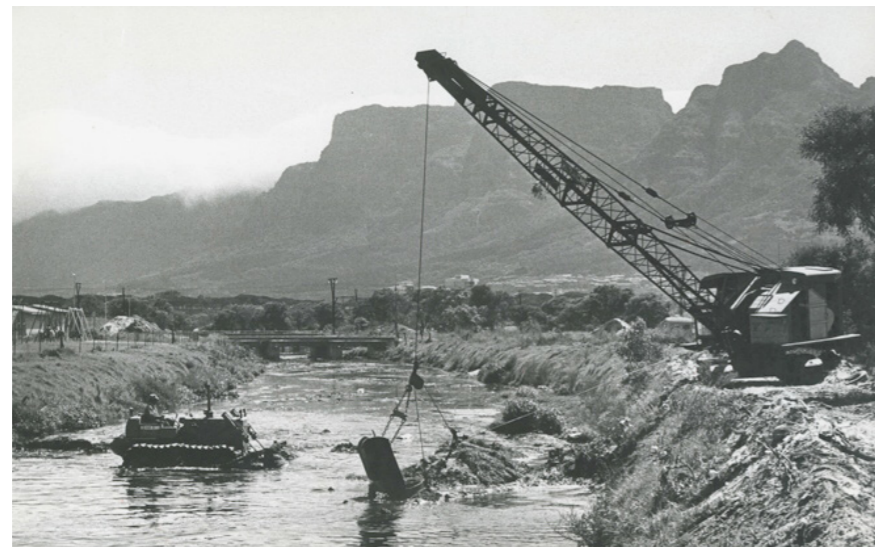
fig. 11. Dredging for the canalisation of the Black River.
