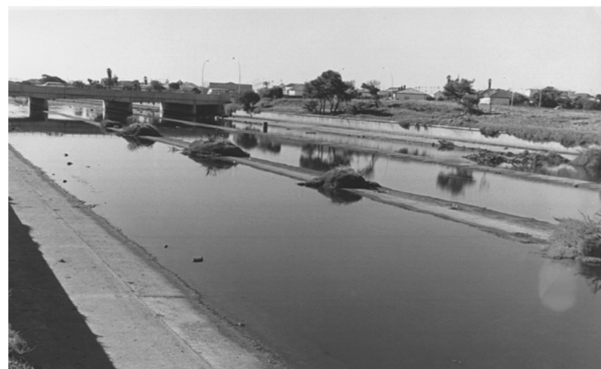
fig. 12. The canalised Black River.
