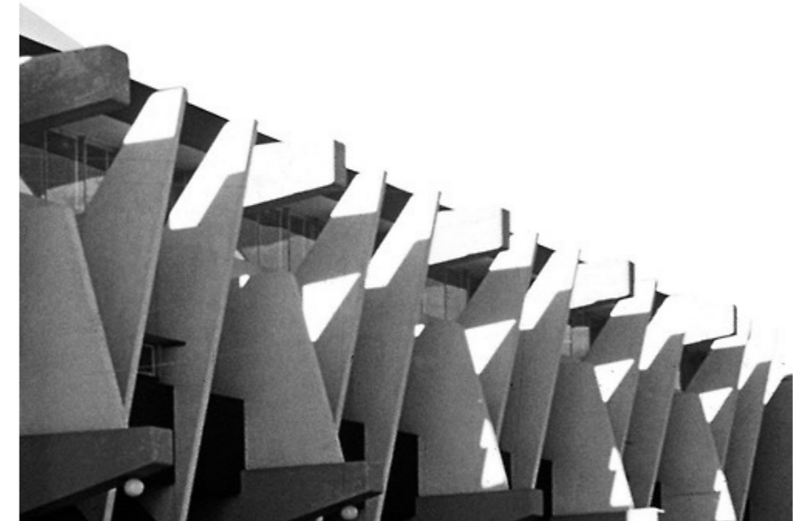
fig. 88. Otto Barbosa office building, 1953 Maputo, Pancho Guedes.
