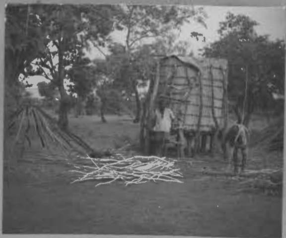
Making a new roof for a maize store
