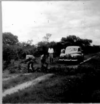
Repairing a washed-out culvert on a reserve motor road
