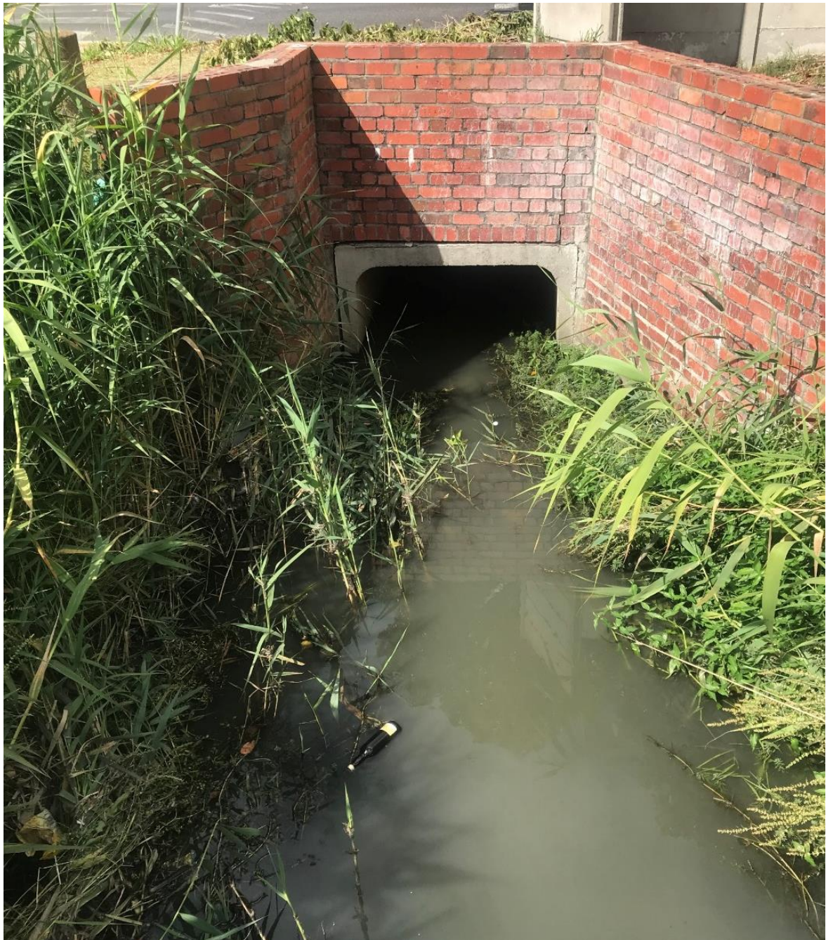
Figure 5-5: The downstream end of the stream behind Blue Route Mall, upstream of its confluence with the Keyzers River
