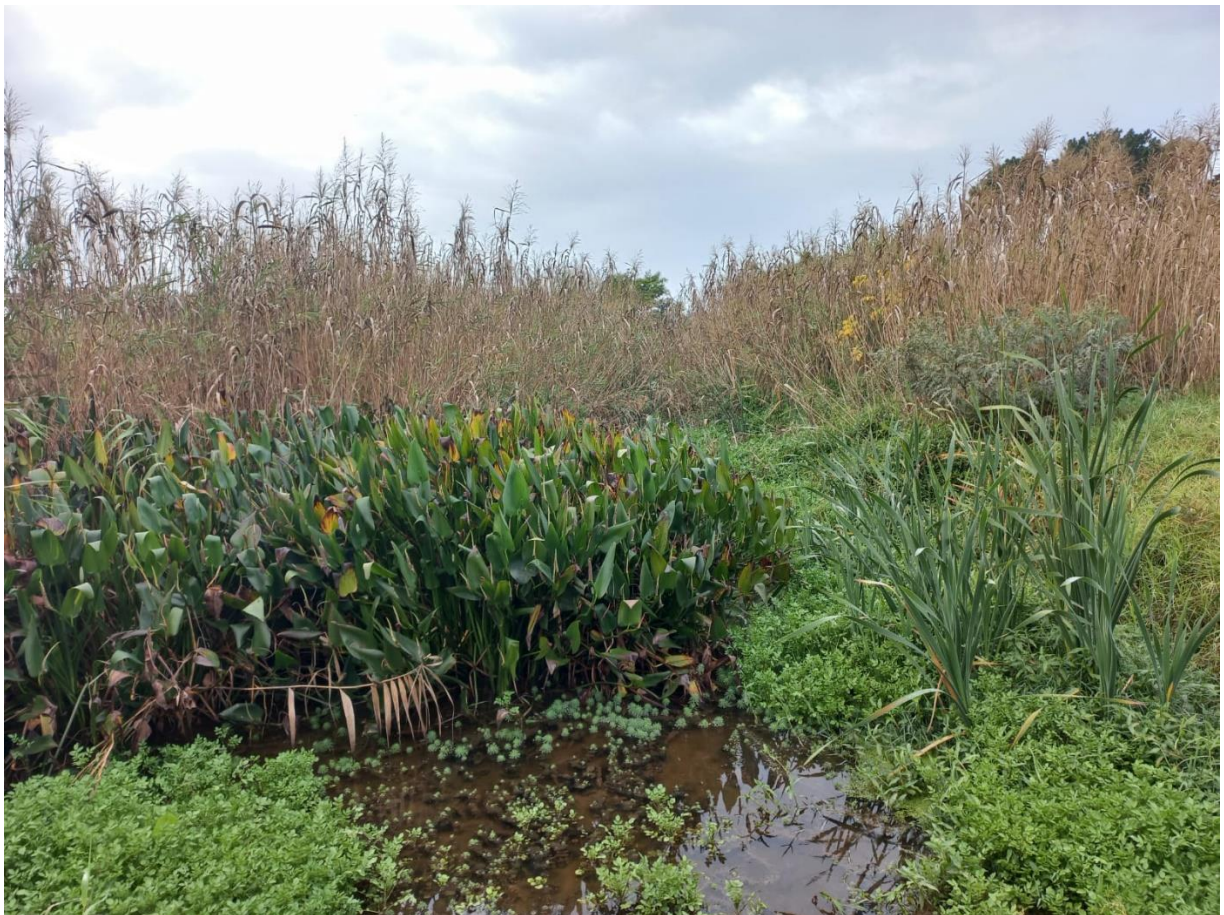
Figure 4-6: The Keysers River just upstream of the M3 culvert. The vegetation growth obscures the view of the culvert (Source: Geordie Thewlis)
