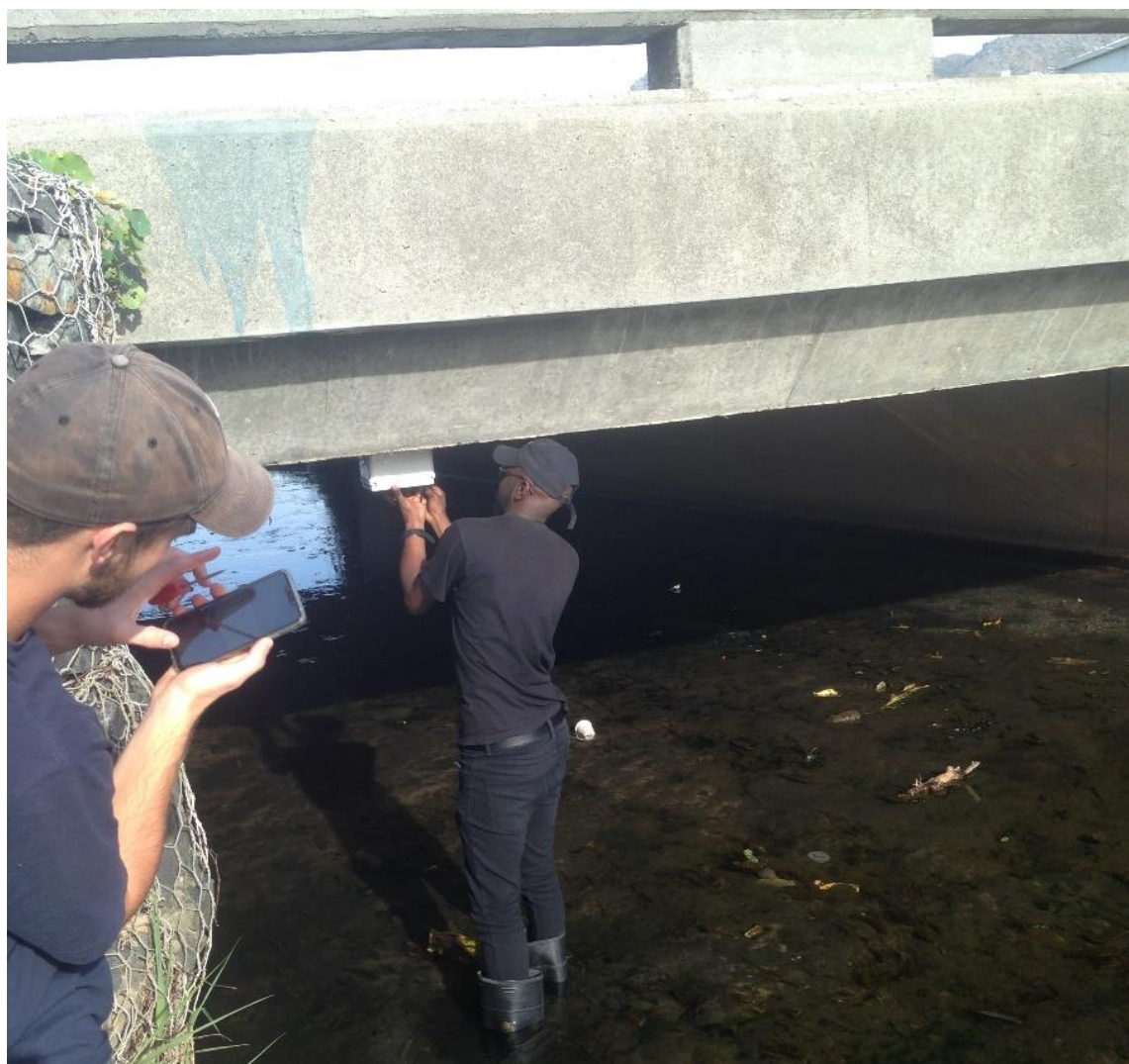
Figure 4-8: Replacing batteries in the Keysers River level sensor
