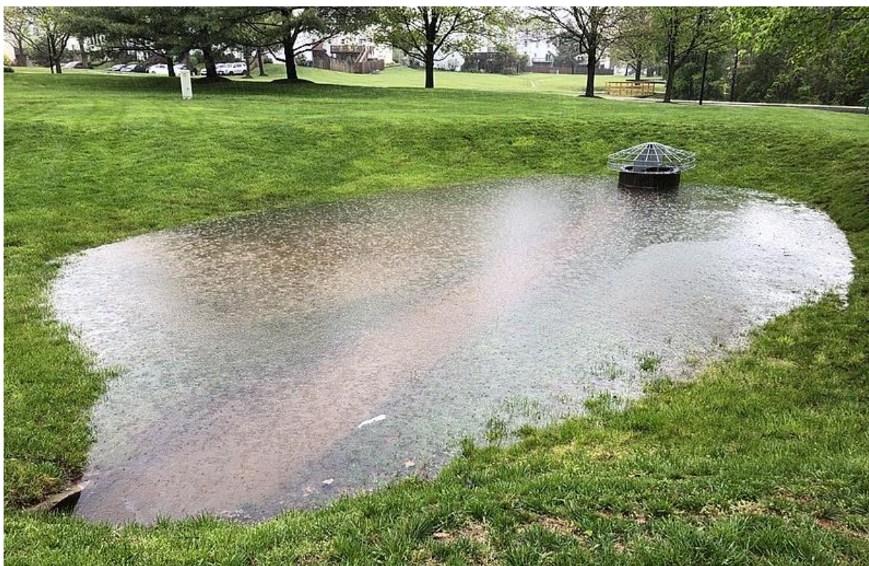
Figure 2-8: Partially filled detention basin during a storm event in Fairfax County, USA (Famartin, 2020)
