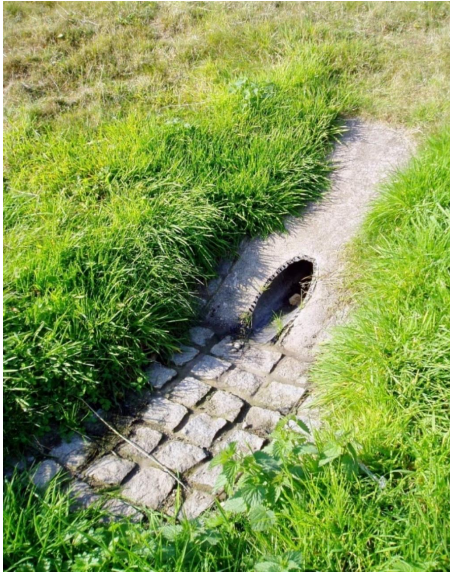
Figure F-2: A typical inlet structure leading into a grassed swale (Susdrain, 2020)
