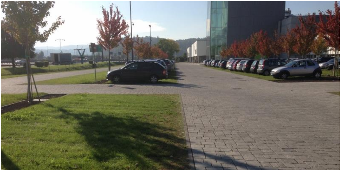
Figure 2-4: Filter strip draining the adjacent paved parking area (CORE, 2020)
