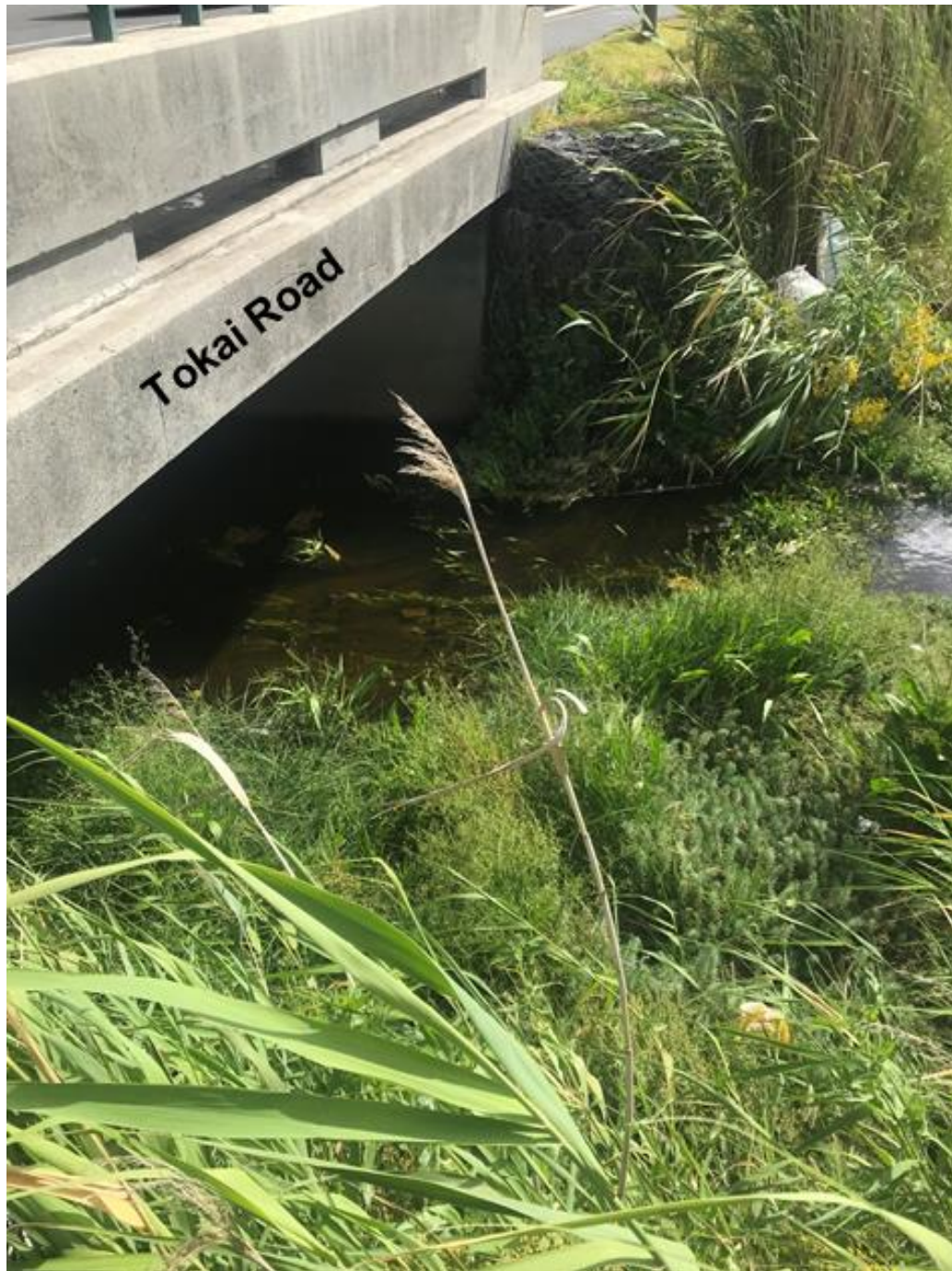
Figure H-2: Site K2, as the Keyzers River flows under Tokai Road (downstream is left)
