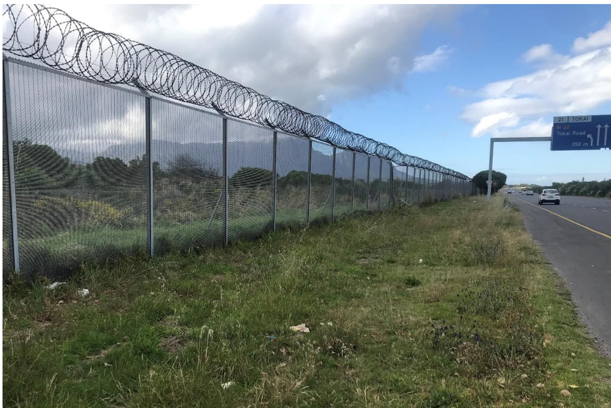
Figure 6-3: Open grass along the M3 freeway with no kerbs along the road
