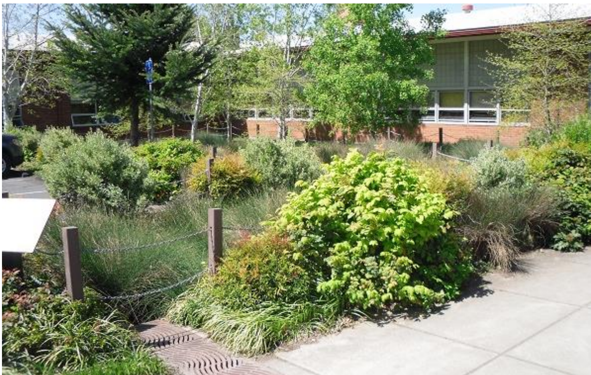
Figure 2-7: A bio-retention system in Portland, USA (EmilyBlueGreen, 2013)
