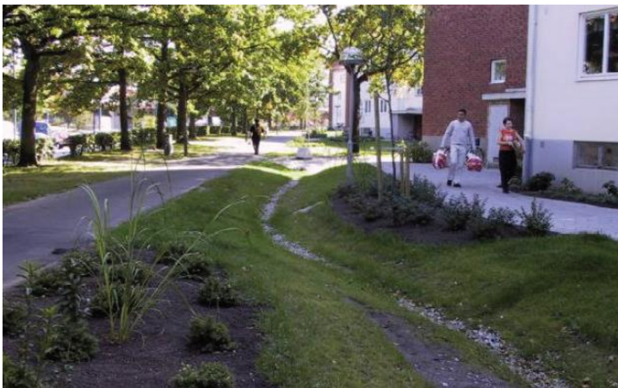
Figure 2-5: A shallow swale in a housing estate in Malmö, Sweden (Wilson et al. , 2010)
