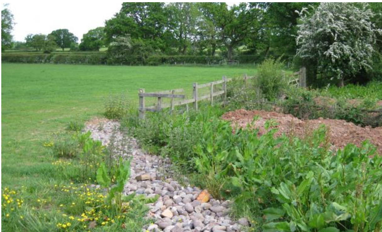
Figure 2-6: An infiltration trench in Warwickshire, UK (Stott, 2010)
