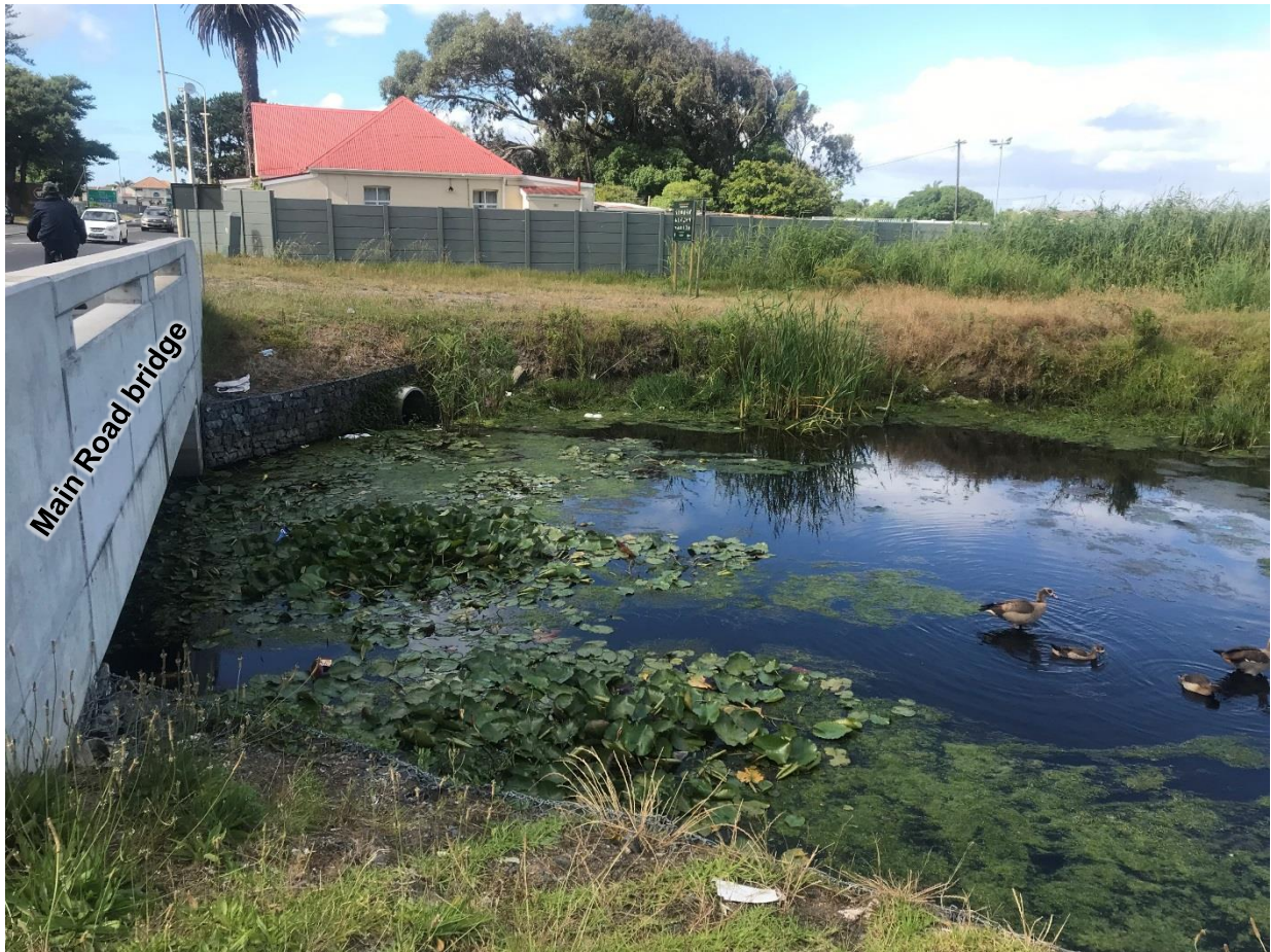
Figure 5-4: Site W6, just downstream of the Main Road bridge (flow towards the right)
