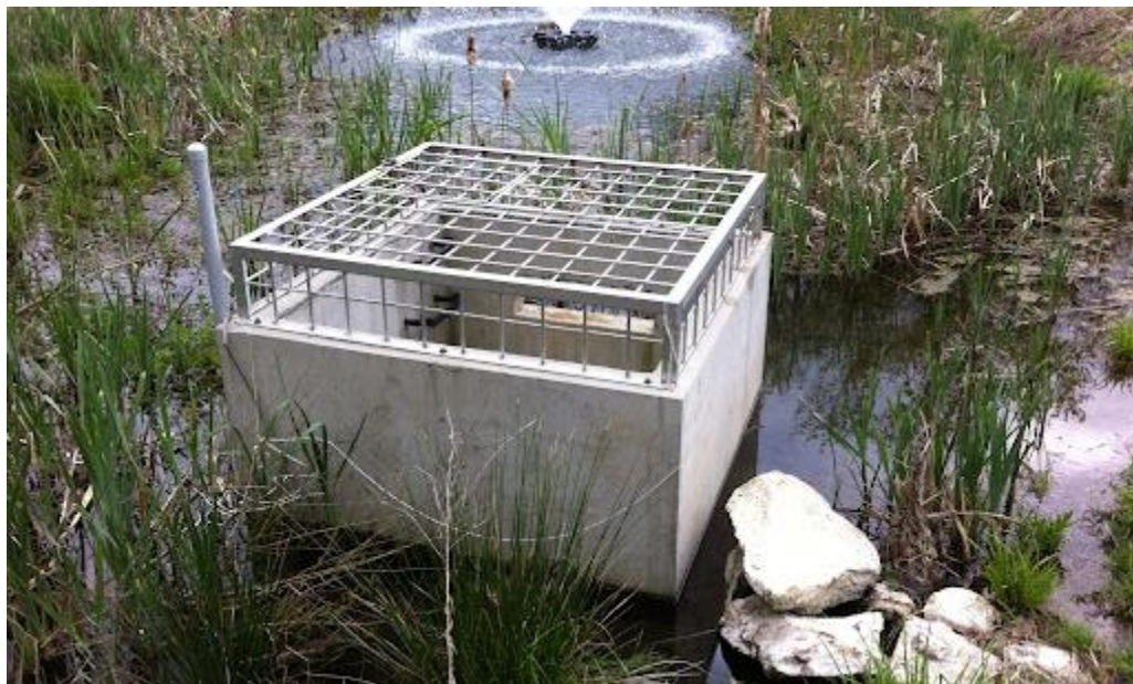
Figure F-4: An outlet control structure in a constructed wetland (SEES, 2021)
