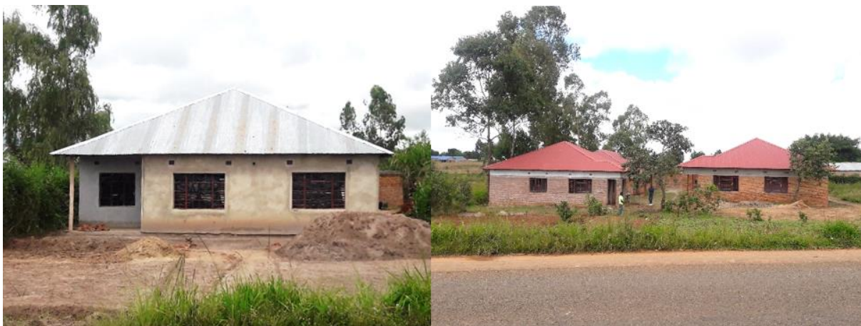
Figure 5.12: Houses Built Despite Agreed Highrise Commercial Zone along Main Road
