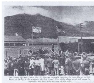
Figure 61: Opening of the Salt River Market. Shed like structures are seen which appear to have been closed up in today's market. Cape Times, 11 December 1939.
