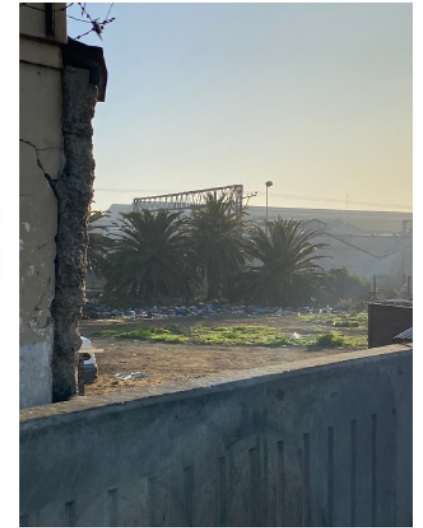
Figure 28: Voortrekker road dead end to the East of the site.
