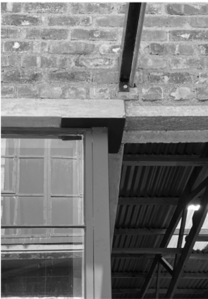
Brick, concrete and steel Figure 102: Reflection and anonymity. Author's own.
