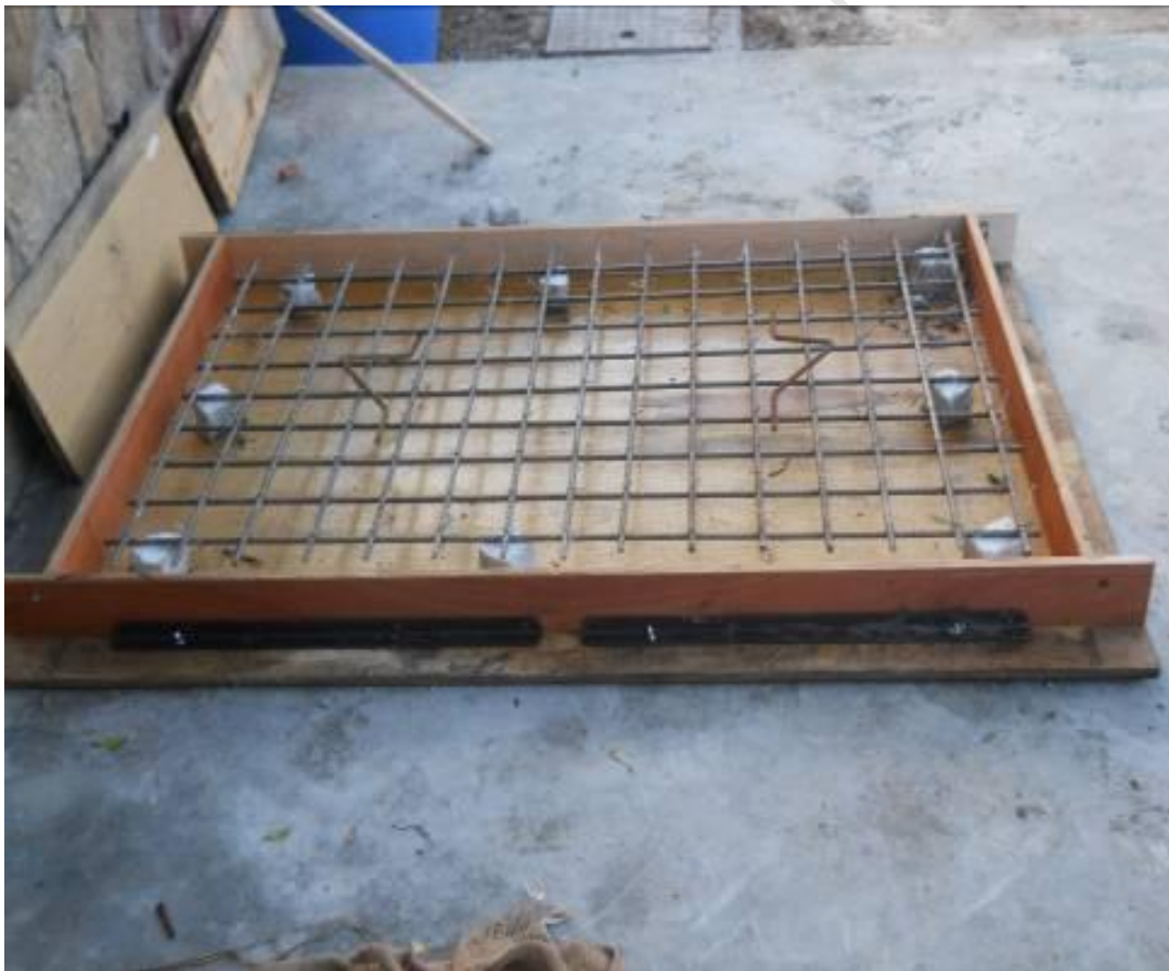
Figure 4.5: Typical mould assembly and rebar arrangement
