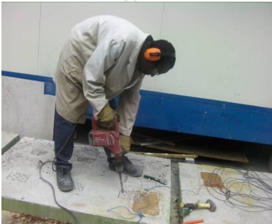
Figure 4.9: Excavation of concrete in preparation for the installation of anodes
