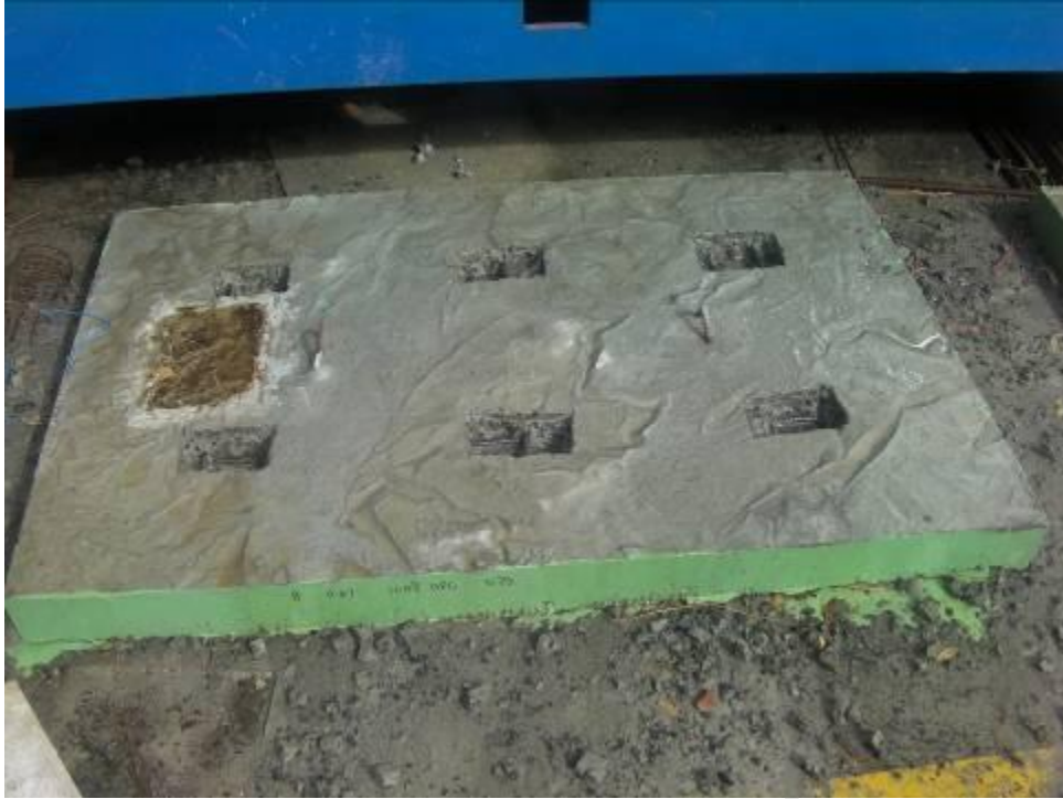
Figure 4.10: Concrete cavities after cleaning with a high-pressure water jet
