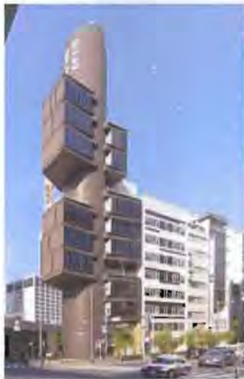
FIGURE 35: Shizuoka Newspaper Co. Building, Tokyo, Kenzo Tange, 1968 (google images) The Metabolists of the 1960s clearly separated vertical circulation along cores and the served space. Many multicore buildings with exposed shafts have been influenced by the Metabolists. Archigram in England envisioned utopian schemes with tall cores
