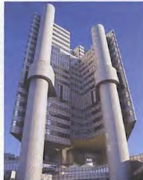
FIGURE 34: Hypobank, Munich, Walter and Bea Betz Architects, 1981 (google images) The 21 storey building features four cylindrical towers connected with a storey high girders on the 11th floor (service plant floor), which forms an irregular outrigger system. This primary structure supports the 15 storey structure above and the hanging 6 storey portion below.
