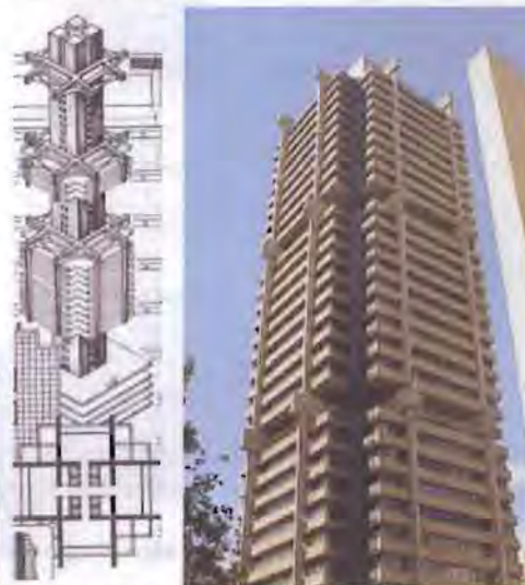
FIGURE 36: Standard Bank Centre, Johannesburg, Hentrich-Petschnigg and Partners, 1968 (Schueller, 1996) Four coupled concrete tubes form the central core, off which storey high concrete beams cantilever at three levels of the building. They support a stack of ten floors each, connected with eight prestressed concrete hangers which carry the vertical loads in tension. This building is a fine example of a concrete suspension structure, using a core and outrigger system showing a high degree of sophistication for its time.
