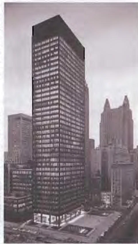
FIGURE 33: Seagram Building, Chicago, Mies van der Rohe, 1958 (google images) The steel rigid framed tube structural system was characteristic of the cartesian skyscraper which was dominant in North America in the 1960s and 70s. The Seagram building is a prime example of this tall building type. The exposed steel frames in this case are however decorative as the load bearing steel had to be covered for fireproofing
