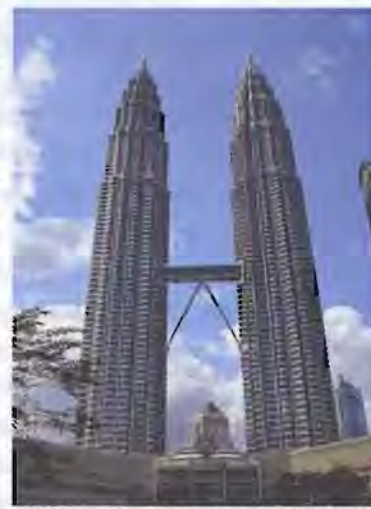
FIGURE 11: Petronas Towers, Kuala Lumpur, Cesar Pelli 1998 (google images) The twin towers represented the idea of a mega-skyscraper, a city within a building.
