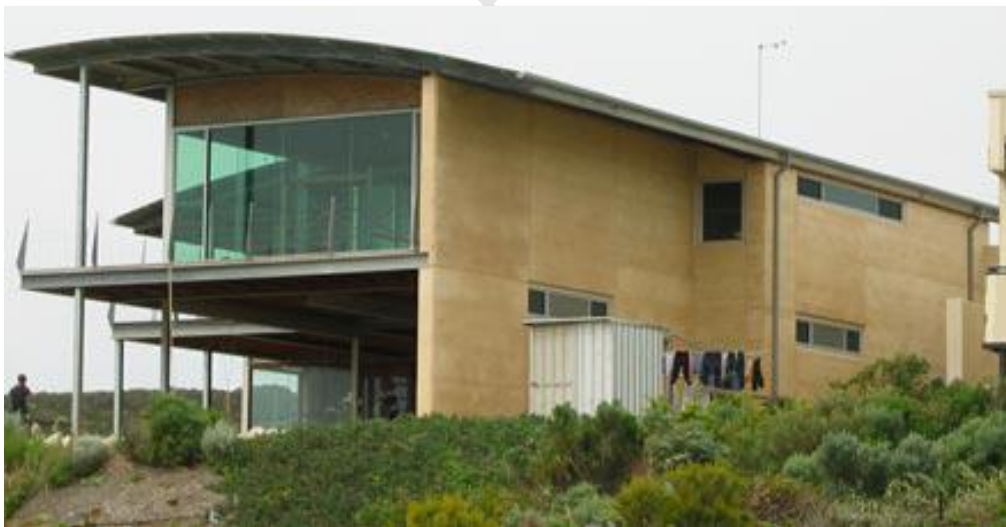
Figure 2.4: Stabilised Rammed Earth house, Western Australia (Walker et al. 2005)
