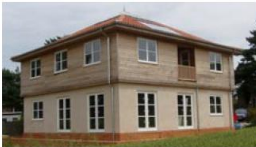
Figure 2.3: Jasmine Cottage built from Stabilised Rammed Earth, Norfolk (Walker et al. 2005)
