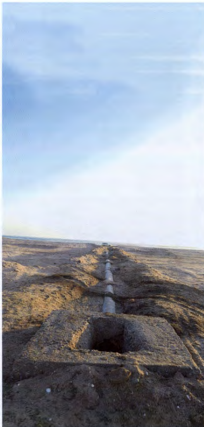
Site: view from pump station mound to sea
