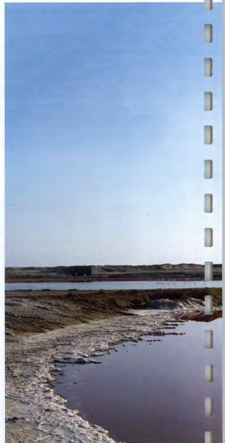
Site: view of existing pump station- from pans to the sea
