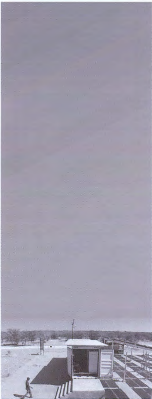
Cuve Waters HD solar desalination plant, Akutsima Namibia
