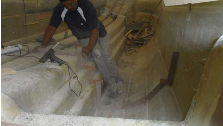
Photo 2: Fitting the bulkhead template
