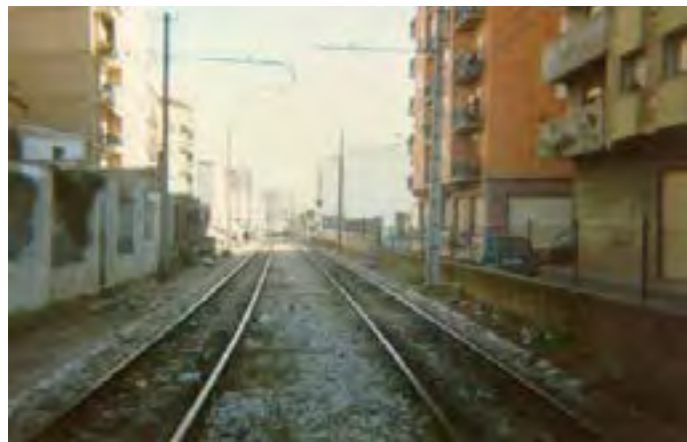
Figure 74: Valencia, Calle Monduber, Railway as barrier. Source: http://siteresources.worldbank.org/INTURBANTRANSPORT/Resources/conversion_rail_lines_pwc.pdf
