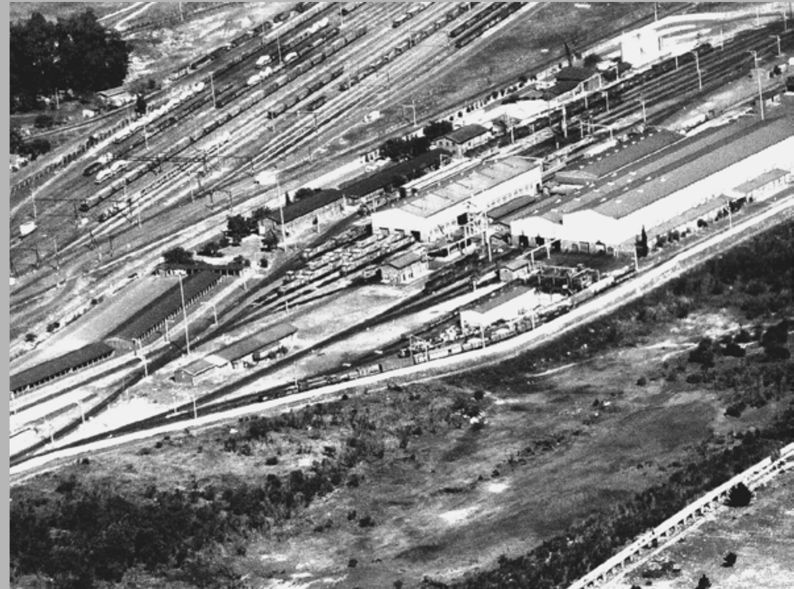
Figure 1: Aerial Photo of Bellville Marshalling Yard, Belcon Site, Bellville.
