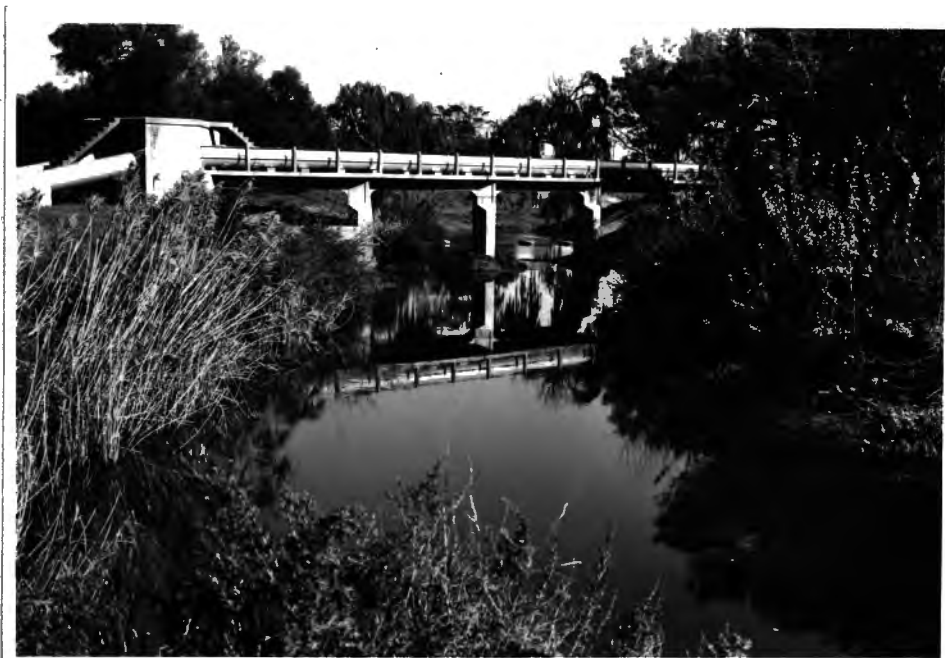
PLATE 8: The Faure Weir on the Eerste River after winter floods. (October, 1976)
