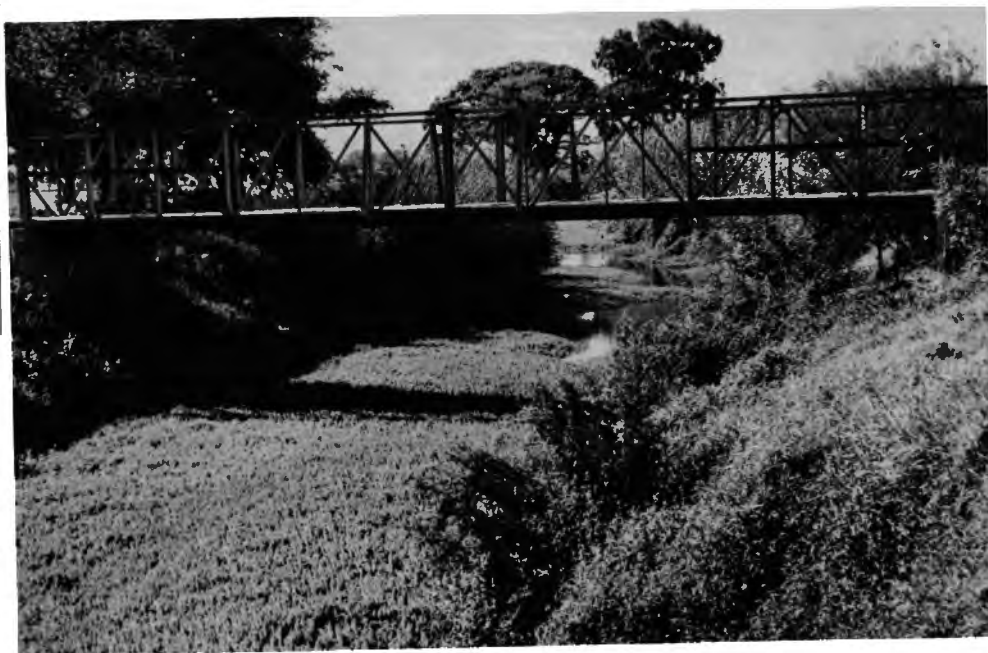
PLATE 9: The Eerste River at Faure prior to winter flooding. (April, 1977)
