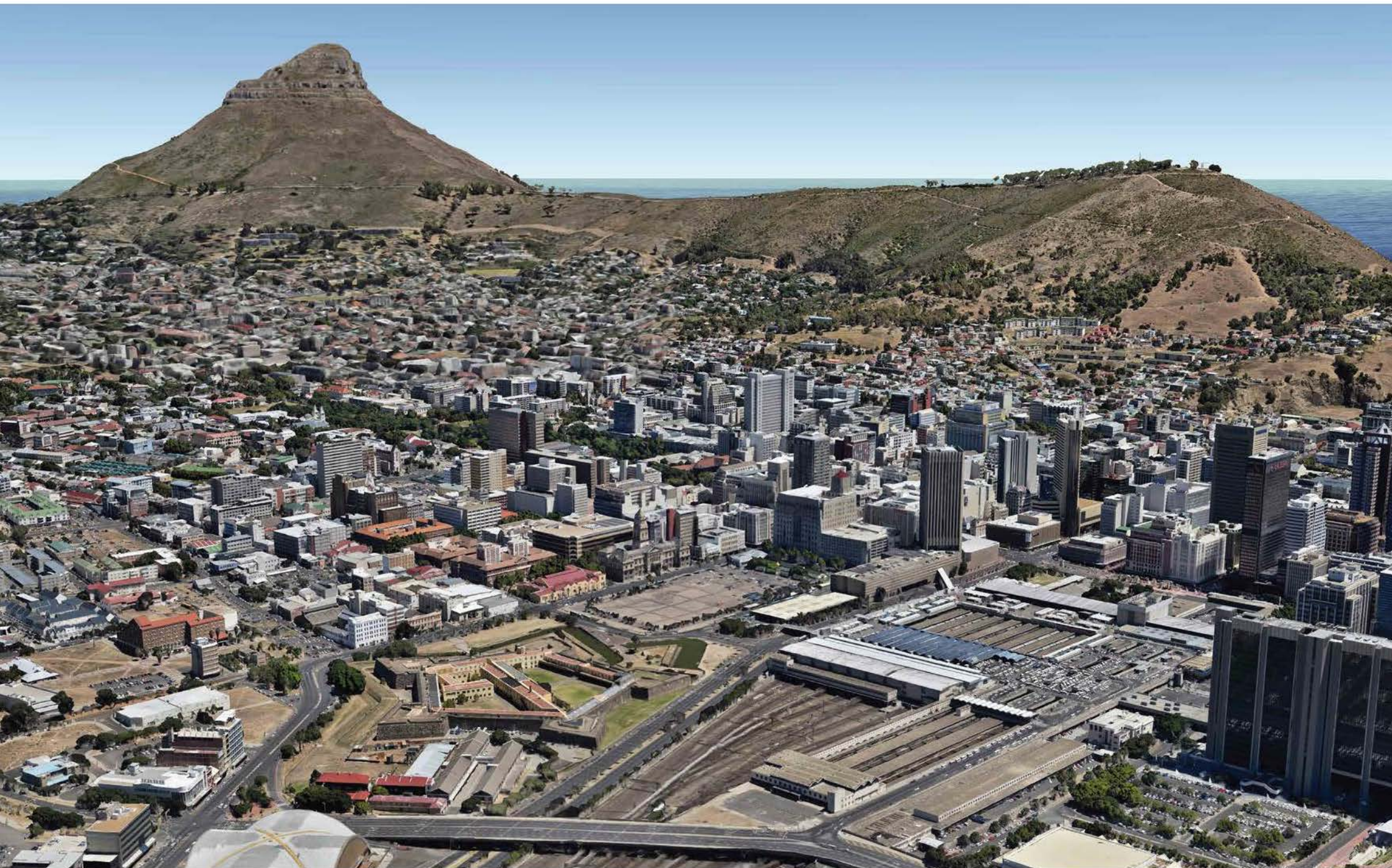
Figure 1.1: The Grand Parade in the context of the Cape Town city centre - Grand Parade at centre (Source: Google Earth, 2017)
