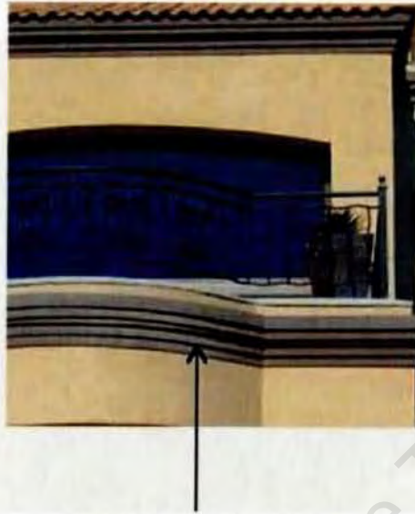
Cladding on a building
