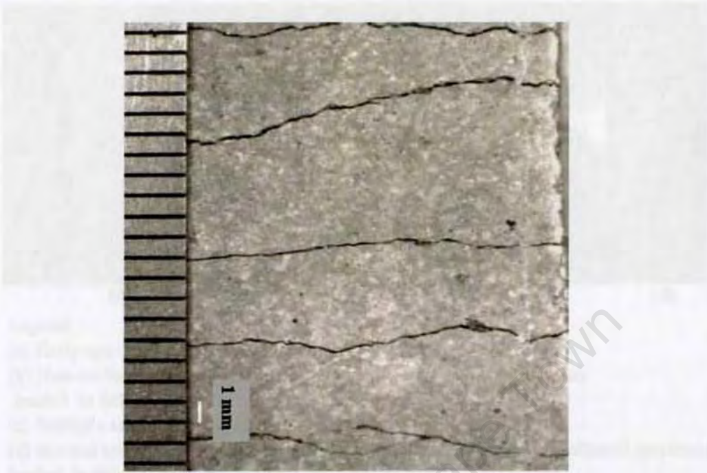
Figure 5.50: Typical multiple cracking at strain hardening stage
