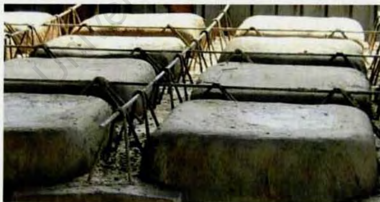
Figure 1.4: Permanent shuttering forms
