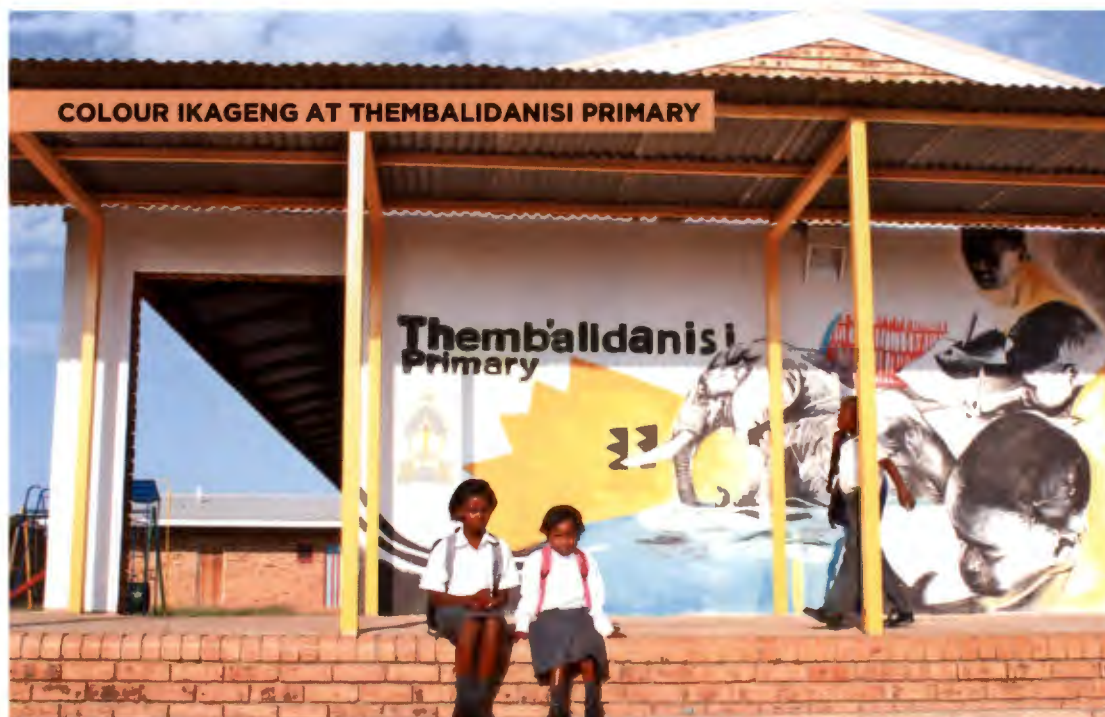
Figure 18: Colour Ikageng finished exterior. Thembalidanisi Primary School, Potchefstroom, 2014. (Colour Ikamva 2015).
