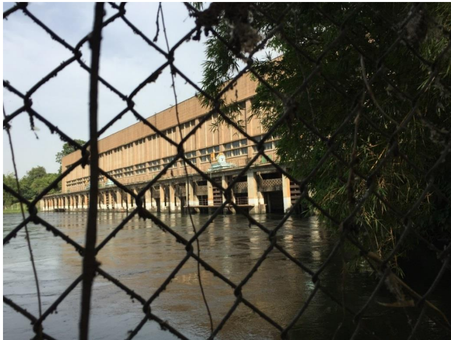
Figure 3.2: Downstream view of Nalubaale Hydropower Plant
