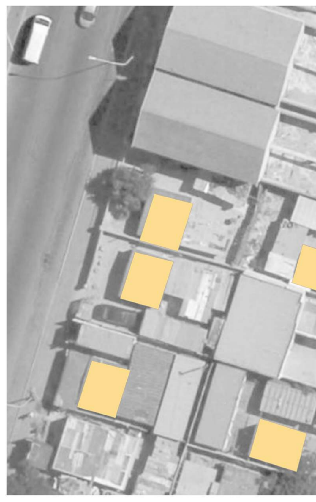
existing RDP self-built additions
