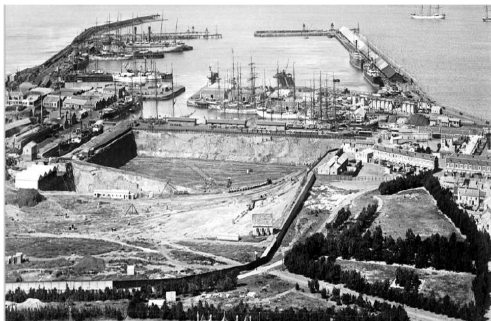
Figure 19: Image of the Cape Town dock in 1912 by "G.B.". The docks in barracks are visible along the central right end of the image (Rennie, John, Teresa Louw, and Gregg Goddard. 1978. The Buildings of Central Cape Town . Cape Town: Cape Provincial Institute of Architects Volume 3).
