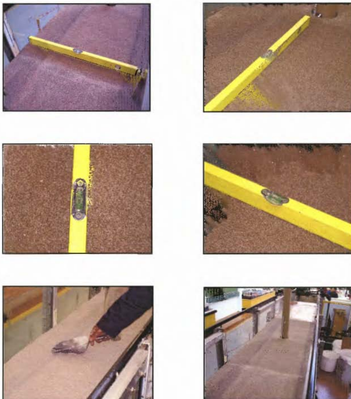
Figure 4-12: Placement and levelling of sand
