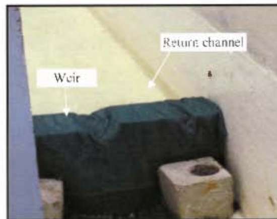
Figure 4-5: Weir in return channel
