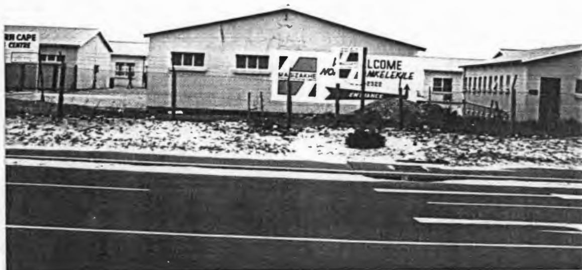
Figure 4.4 Masizakhe as seen from the main access road to WCTC
