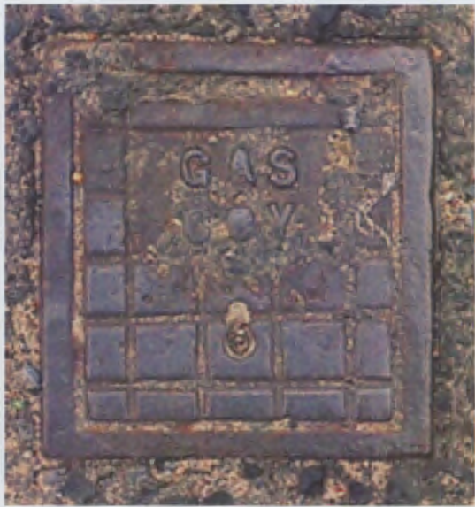
Figure 42 Typical gas company inspection plate, 2001.
