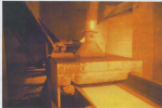
B251: bottom of hopper on track 3 serving intake elevator #1.
