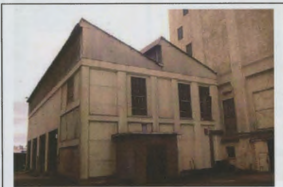
Figure 80 Cape Town: the hydraulic accumulator house, 1995.
