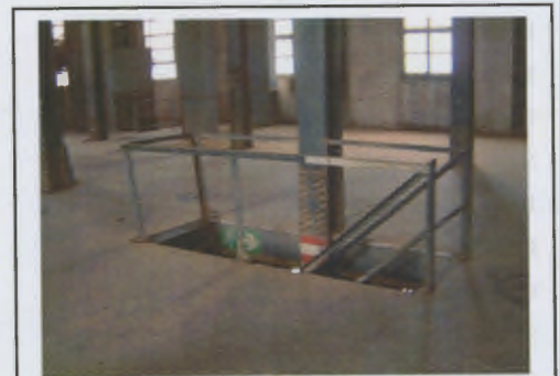
B066: steel stairway to cross belts on level 1C.
