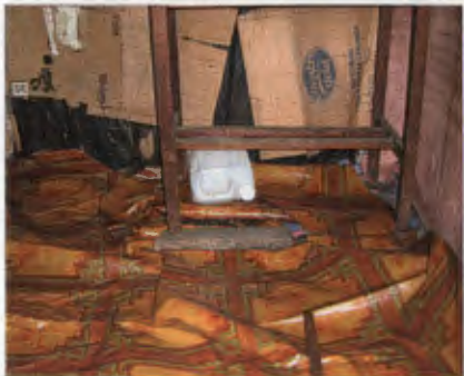
Figure 109: mitigation: layers of sheeting on floor
