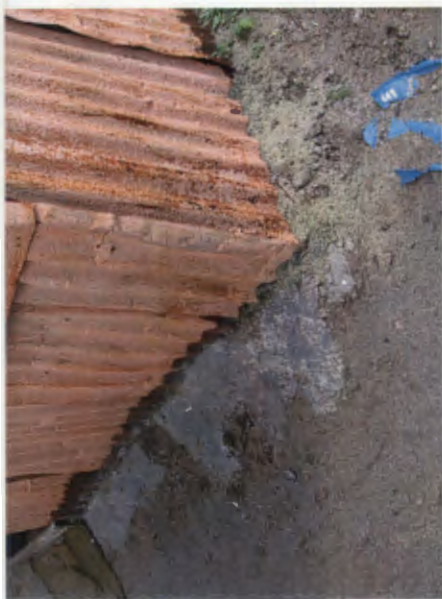
Figure 110: mitigation: cement around edge of shack
