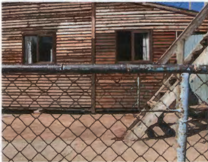
Figure 108: mitigation: day-care raised from the ground
