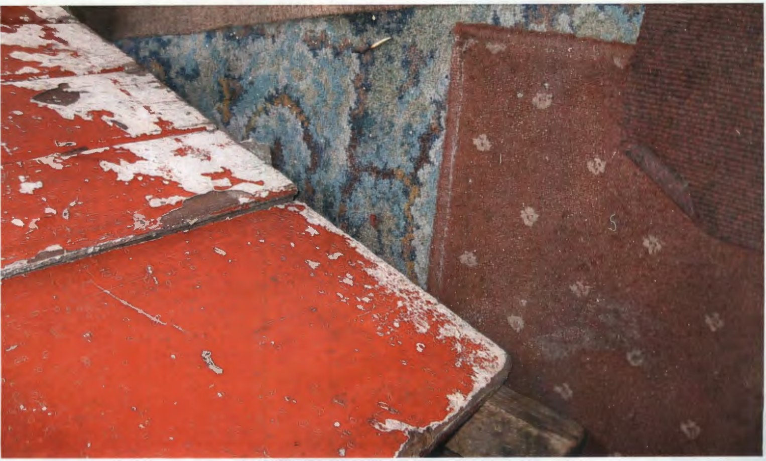
Figure 116: mitigation: layers of flooring
