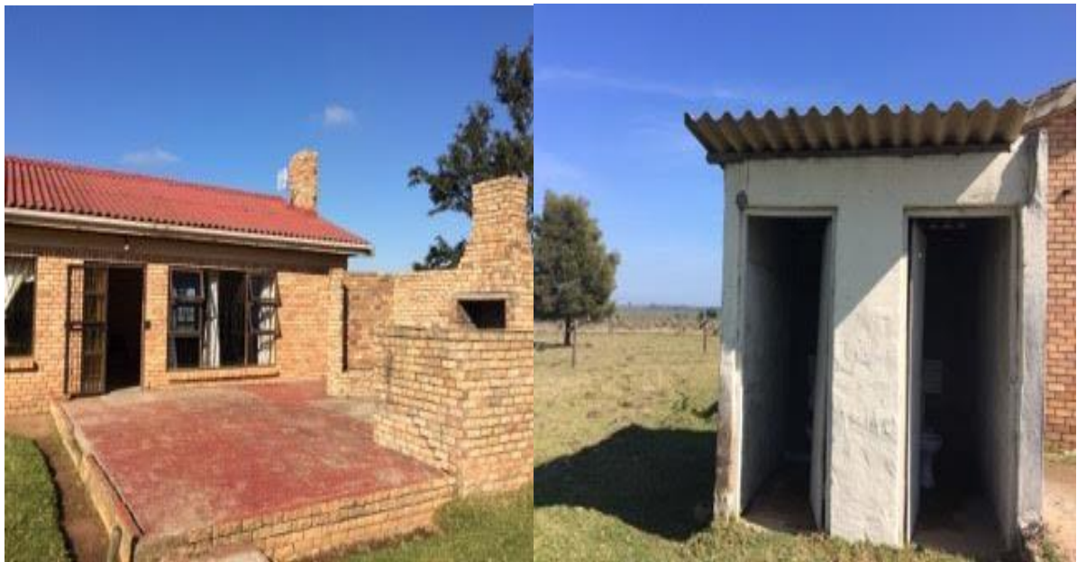
Figure 16: The TDT office and its outside toilet. (Photo by the author, 2017).
