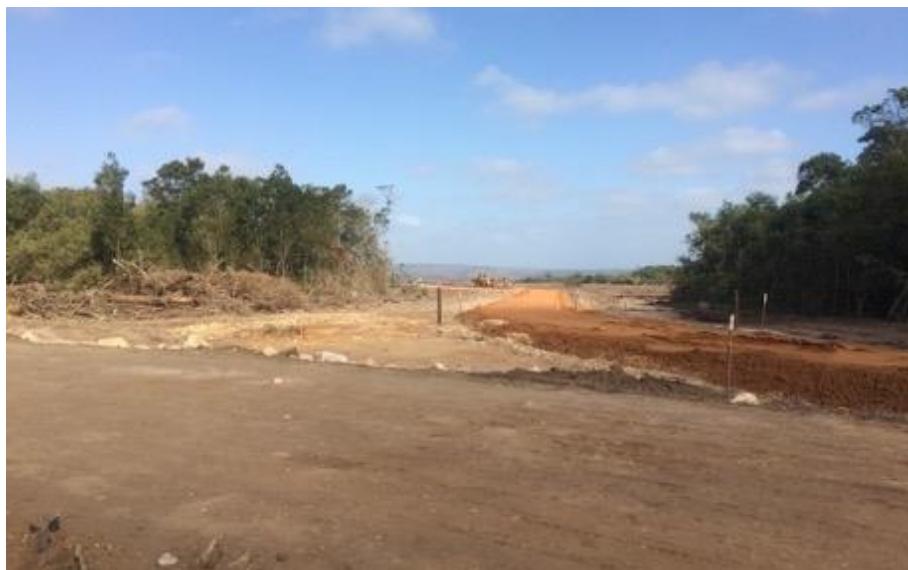
Figure 8: Tsitsikamma Community Wind Farm under construction. (Photo by the author, 2015).
