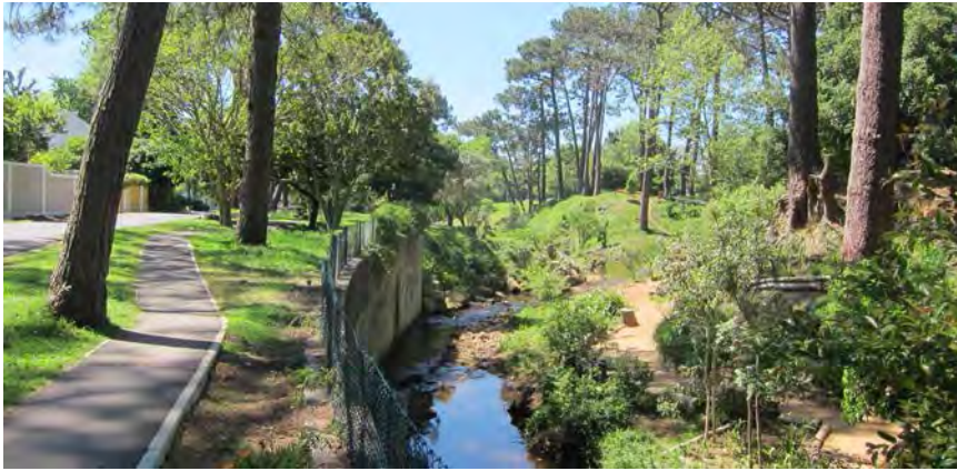
Figure 4.13: a photograph of the upper Liesbeek River Corridor which is a hybrid canalisation system that includes a well-developed riparian buffer with sufficient vegetation and pathways to encourage recreational activity to enjoy the river environment (Author's Own).
