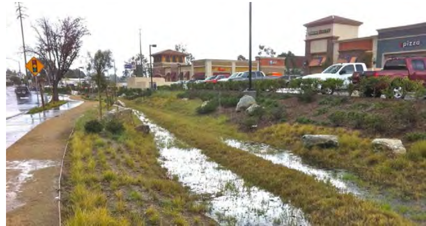
Figure 5.6: A photograph of a Bio-swale that is harvesting and filtering stormwater from the surrounding road network and car park, located in the United States of America (MHA Group, 2012).
