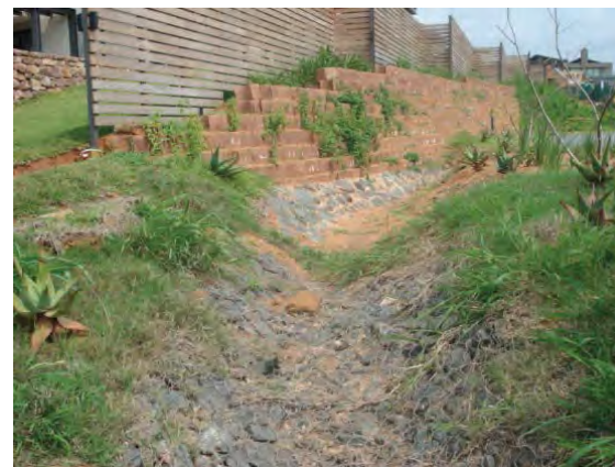
Figure 5.7: A photograph of a Bio-swale that is harvesting and filtering stormwater from the surrounding road network and residential area, located in Umhlanga, KwaZulu Natal, South Africa (Armitage et al , 2013: 39)
