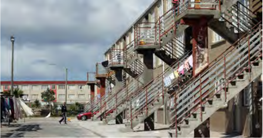
Figure 41: In the Cape Flats Walk-ups, the many unprotected exterior staircases overlook the back courtyard, instead of overlooking the street side to create surveillance. Thus the circulation system is both inefficient and does not create positive community environments.
