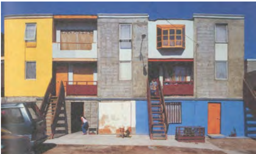
Figure 97: The lightweight board wall allows for easy extensions to the side of the unit.
