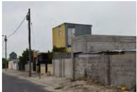
Figure 82: Concrete block double storey renovation.
