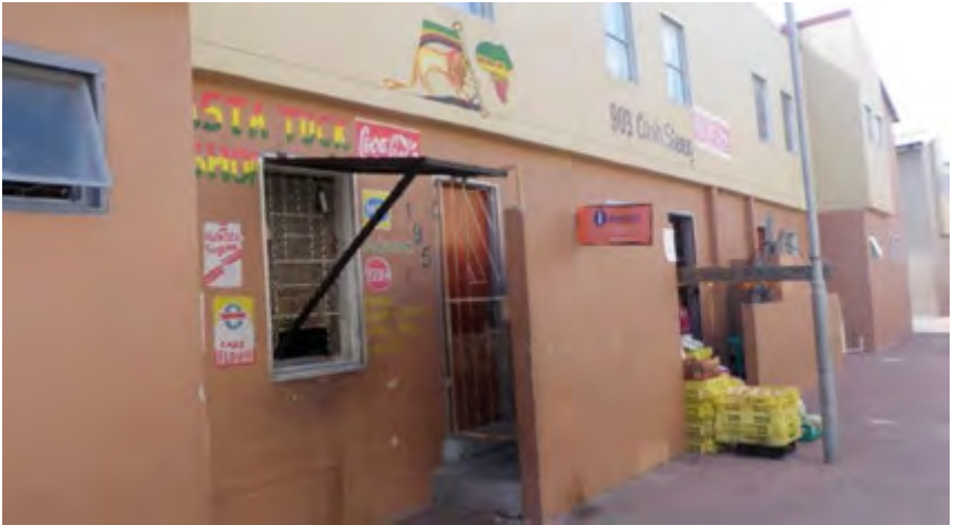
Figure 8: The very tight open space around the units means that mostly very small alterations can be achieved, such as the addition of security fences
