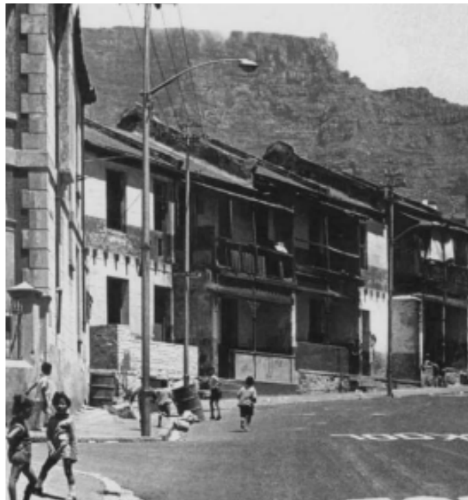
Figure 42: Photo showing stoeps along De Villiers Street
