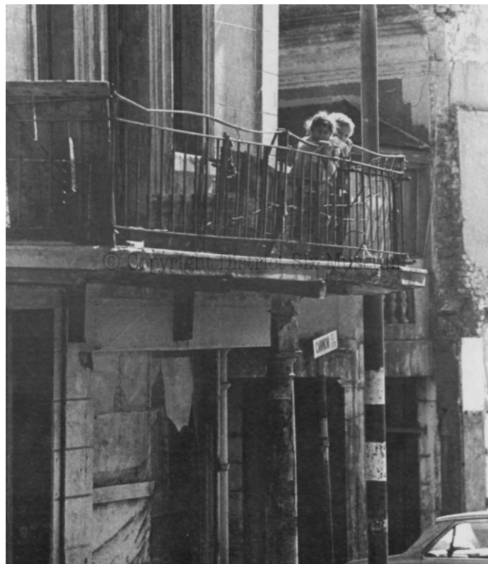
Figure 46: Photo showing the walkway on Canon Street created by the residential balcony above
