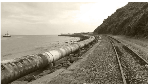
fig. 20 sewage and train infrastructure
