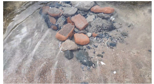
fig. 32 erosive forces present on site
