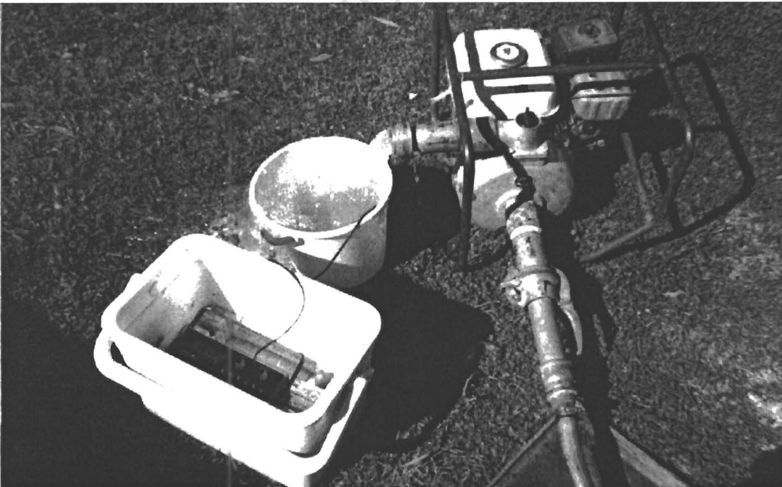
Figure 3.3: Purging the borehole while continually monitoring the electrical conductivity.
