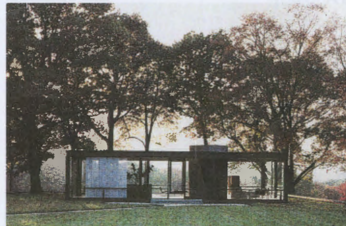
Glass House, New Canaan, Connecticut (USA), by Philip Johnson
