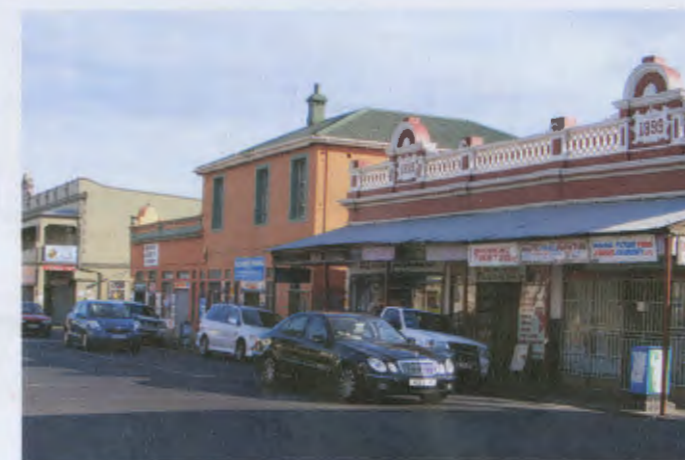
View of site from St Luke's Church
