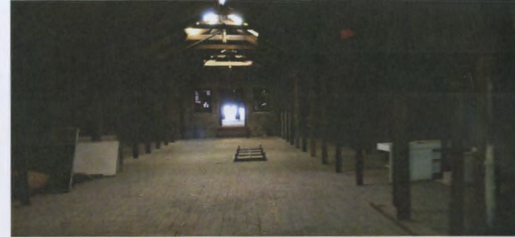
View of attic space of the second half of the building
