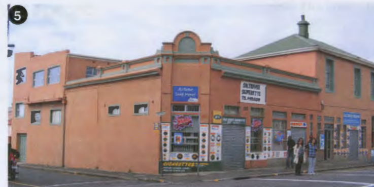
5 Restore Building with a low heritage value situated on corner of Albert and Portland Road [renovations and pedestrian overhand removed]
