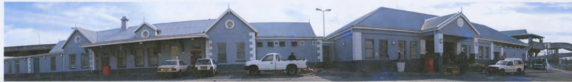
View of Salt River Station in Foundry Road, inhabited by small scale traders during the day
