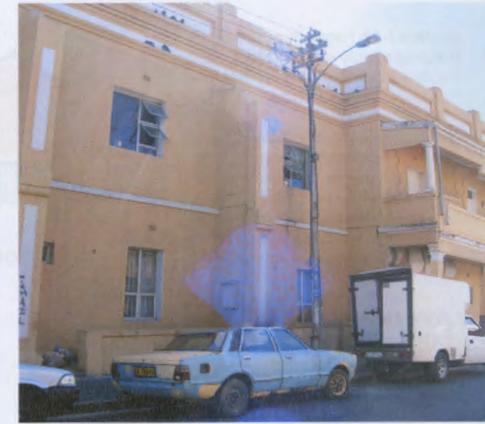
View of two storey apartments in Portland Road.
