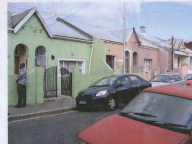
View of row houses in Portland Road
