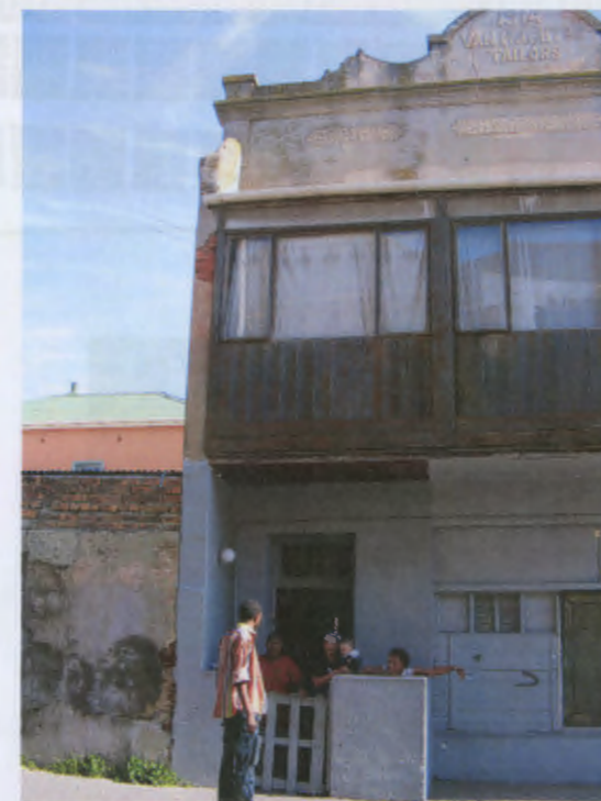
Image of Van Hacht's building adjacent to Lane 2
