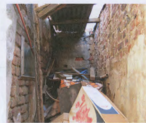
View from Lane 3 looking towards Lane 1
