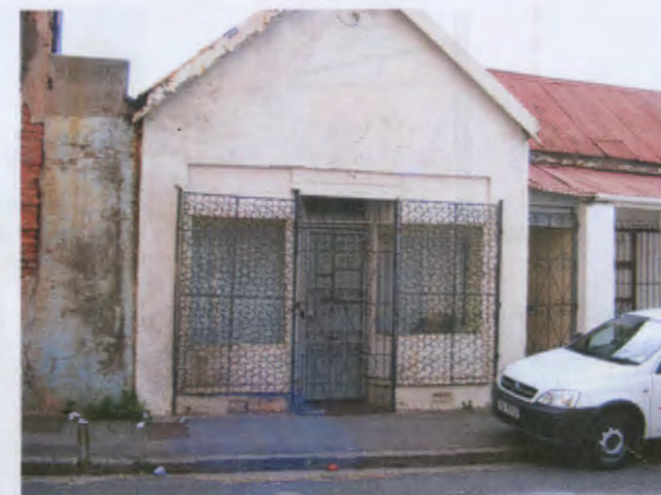
View of Tailor's shop and home
