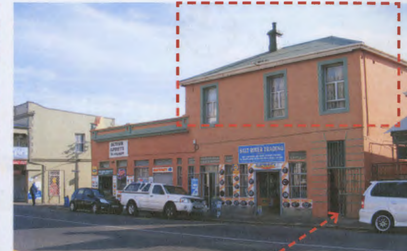
View of building owned by the Hassan Family Entrance to living upstairs [arrow showing entrance]
