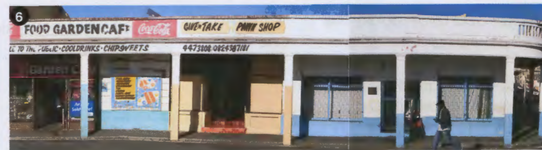
6 Restore Building with a low heritage value situated on corner of Foundry and Pottland Road [upper floors demolished due to aging, decaying structure]
