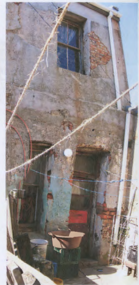
View of adjacent yard [Used by residents on first floor]
