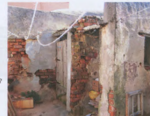
View of outdoor toilet in yard looking towards Lane 1
