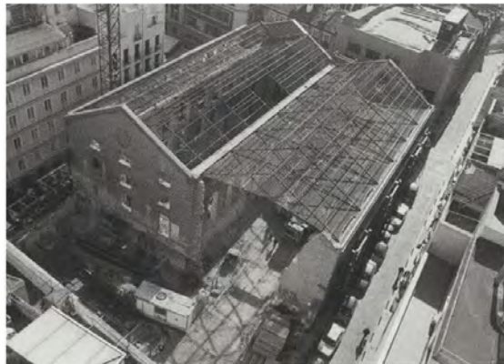
Existing Mediodia power station (Chevrier, 2010: 92)
