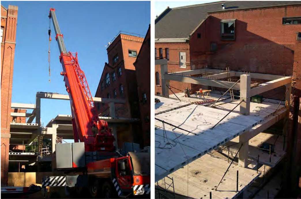
Insertion of precast columns in between two existing buildings (Nastasi, 2010)
