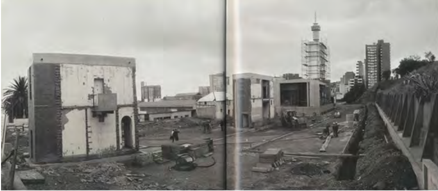
Figure 24: Constitution Square under construction, Awaiting Trial stair towers remained(Law-Viljoen, 2006: 34-35)
