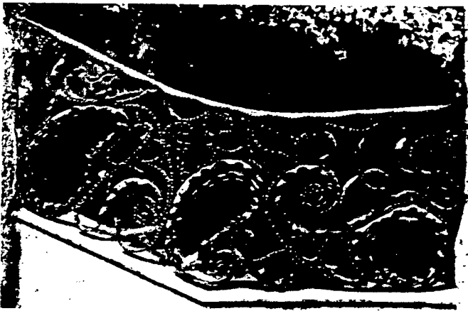
Gaudí: Casa Milá, Barcelona, 1905-10. In the interior the banisters seem like creeping, wreathing seaweed.
