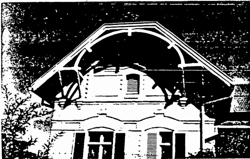
Redecker: 69 Leutweinstrasse, Windhoek, 1906. The decoration consists of small circles on the ends of the brackets supporting the roof and ellipses and straight lines above the windows.
