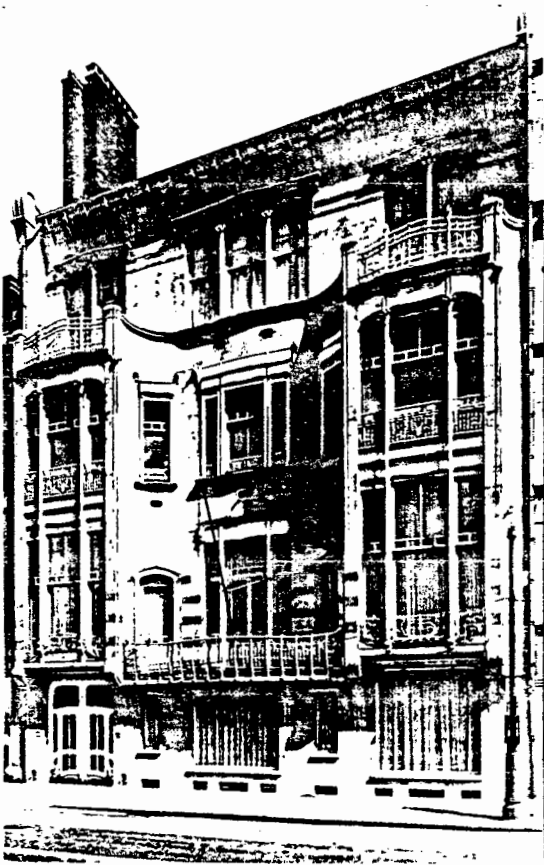
Horta: Hôtel Solvay, Brussels, 1895-1900. The facade displays a markedly plastic treatment and the structural elements are also freely exposed. The interior is an ample expression of flexibility, light and spaciousness.
