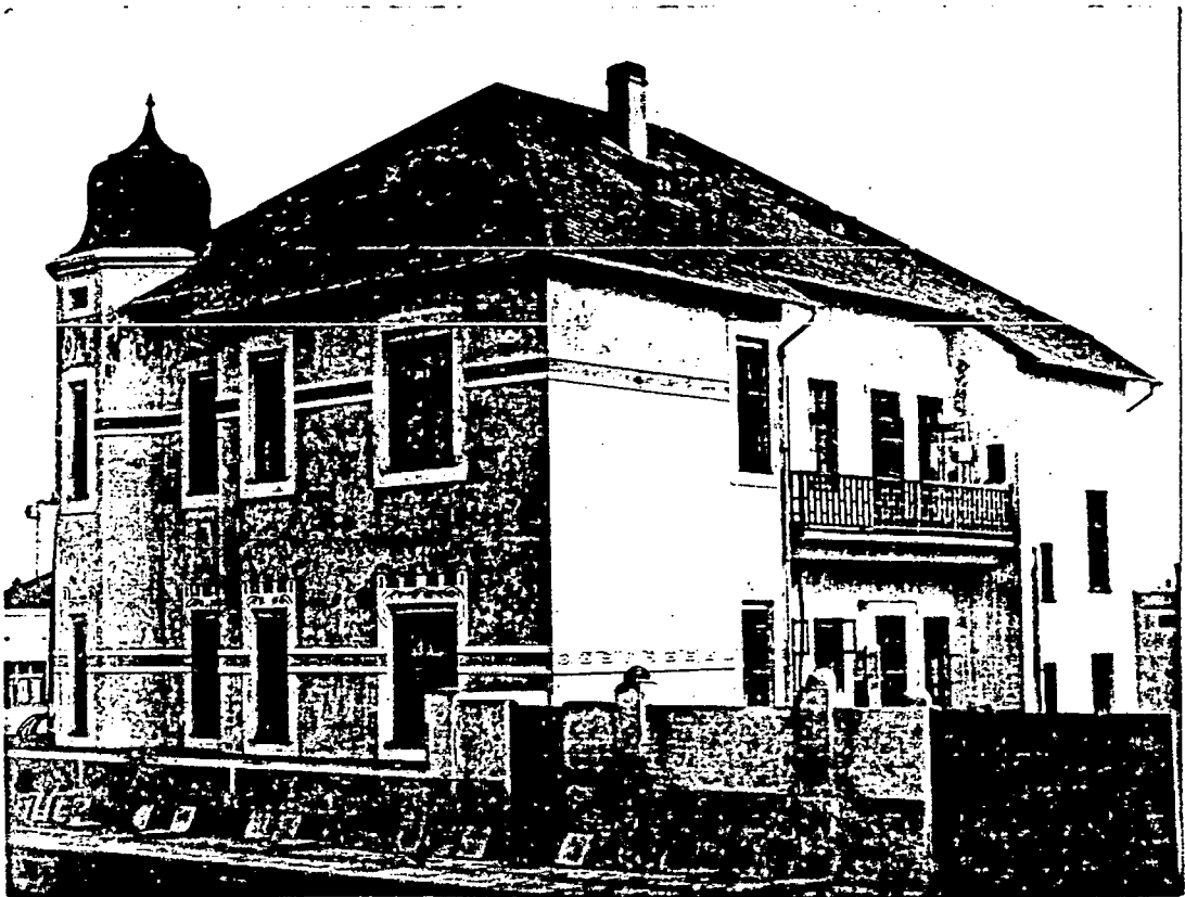
Willa: Haus Wille, Swakopmund, 1904. The frugal use and placing of geometrical ornament, emphasizes both the ornament and the plain surface.
