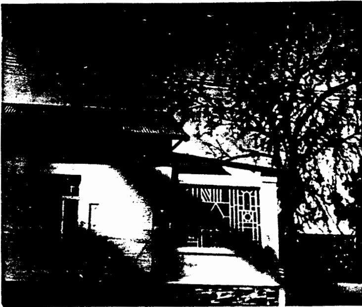
Dwelling corner Post- and Steubelstrasse, Windhoek, 1907. The panes in the rectangular window are asymmetrically arranged and consist of slender rectangles, small squares and circles.
