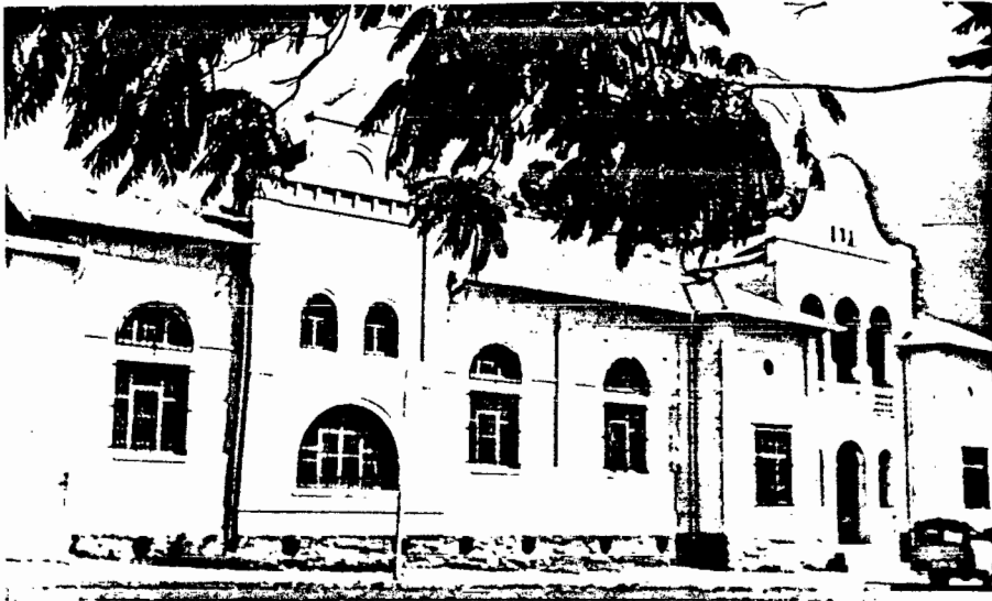
Busch: Turnhalle, Windhoek, 1908, now used by Dept. of Defence. The asymmetric distribution of the windows at various levels creates the impression of a multi-storey building terminated at different levels.
