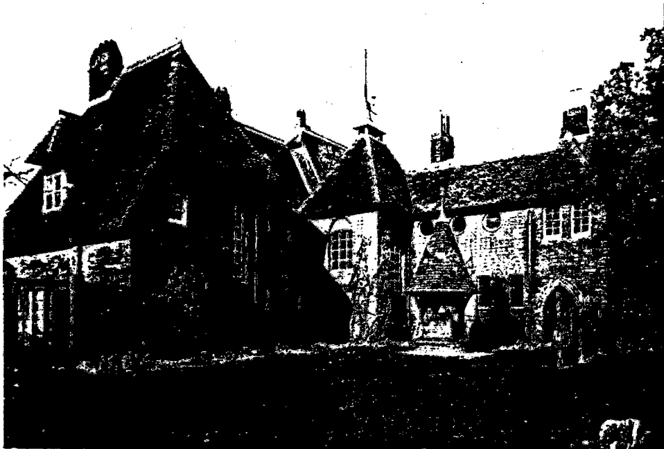
Webb: Red House, Bexley Heath, 1859. Although built for Morris a champion of the Neo-Gothic, the house does not show direct Gothic influence, except for a few arches, but rather expresses the ideals of medieval craftsmanship. Construction is exposed; both in the brick walls on the exterior and in the beams of the ceilings in the interior.
