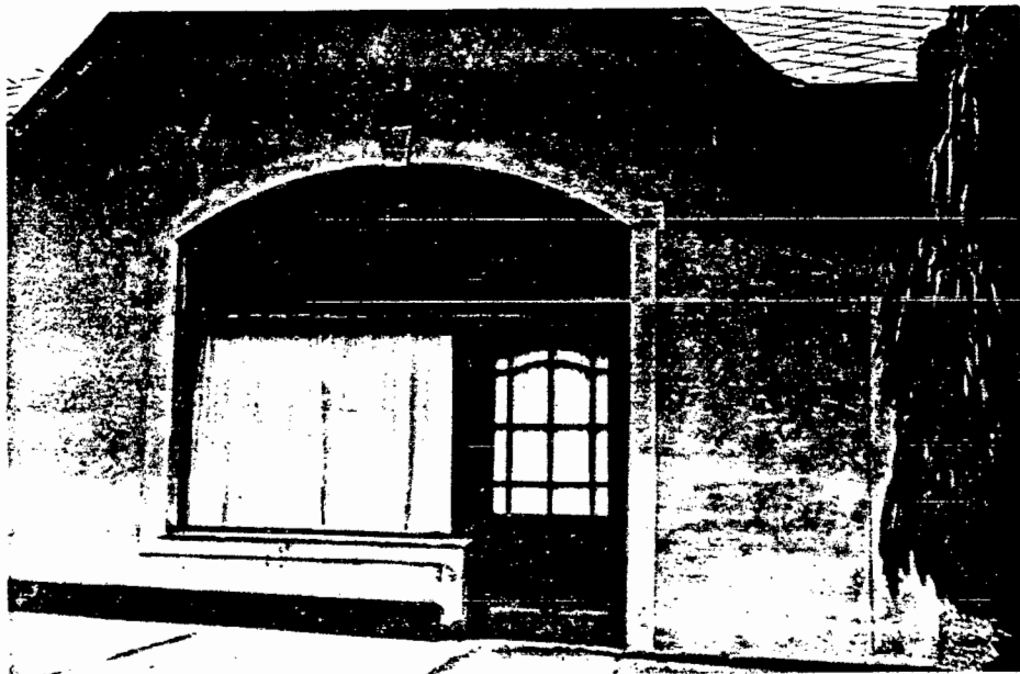
11 Brückenstrasse, Swakopmund, circa 1906. Asymmetry, an essential feature of Jugendstil, is achieved here in the design of the window.
