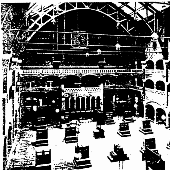
Berlage: Stock Exchange, Amsterdam, 1898-1903. In the main hall the construction of the roof is exposed and the character of the unadorned surfaces emphasized.
