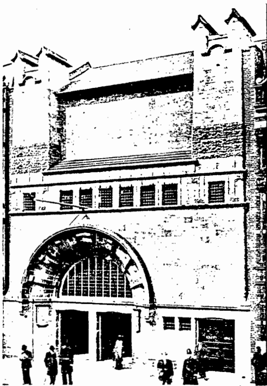
Townsend: White Chapel Art Gallery, London 1897. Basically a symmetrical unit, but with a dynamic plastic treatment, an asymmetrically placed entrance and geometrically abstracted ornament.
