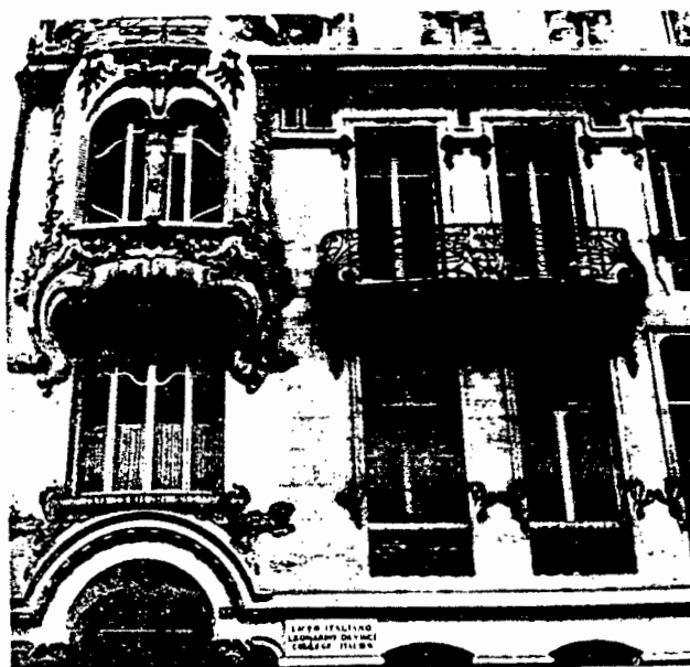
Lavirotte: 12 Rue Sédillot, Paris, 1899-1901. The facade treated with ceramic tiles forms a decorative unity. In the plant-forms draped around the windows and in the balcony railings, the pliant qualities of Neo-Baroque are blended with Art Nouveau.
