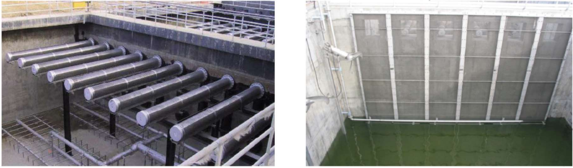
Figure 12.1: Retaining sieves for biofilm carriers that prevents loss of carriers. The sieves require a large surface area to keep approach velocities to a minimum, preventing fouling of the sieves by carriers.
