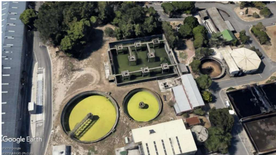
Figure 13.1: Aerial view of the Borchers Quarry A-Works before being upgraded.
